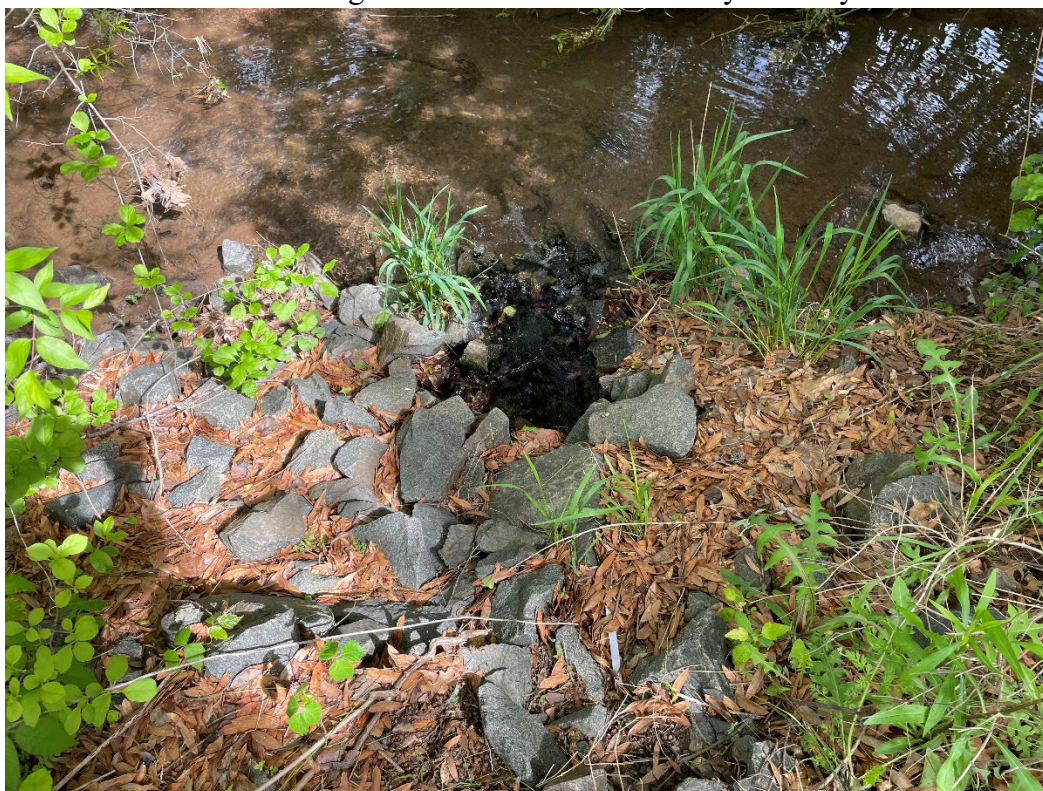
Photo #4. Treated effluent discharges into the unnamed tributary to Stony Brook.
