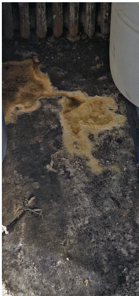
Figure 3 - Another photo of freestanding water and various chemical residues and powders observed within the hot room in-storage area.
