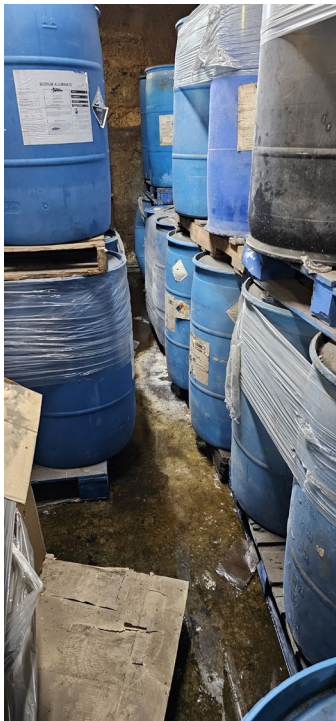
Figure 1 – Freestanding water and various chemical residues and powders observed within the hot room in-storage area.
