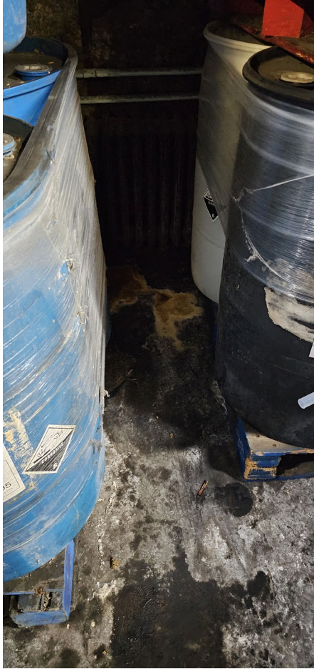
Figure 4 - Another photo of freestanding water and various chemical residues and powders observed within the hot room in-storage area.
