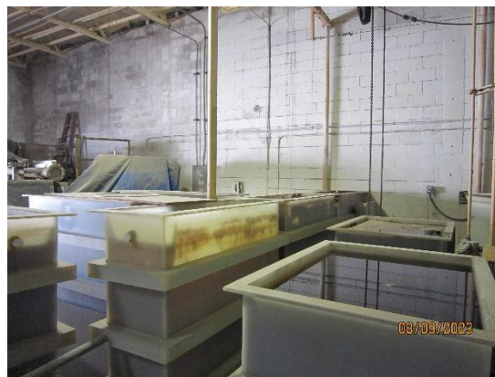
Photo #16 – Plating waste stored in the poly tanks.
