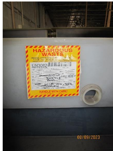
Photo #18 – Plating waste stored in the poly tank.
