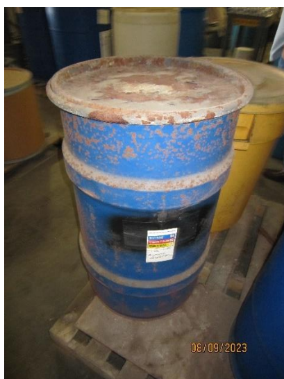
Photo #23 – Rusted container of aluminum sulfate in the chemical storage area.
