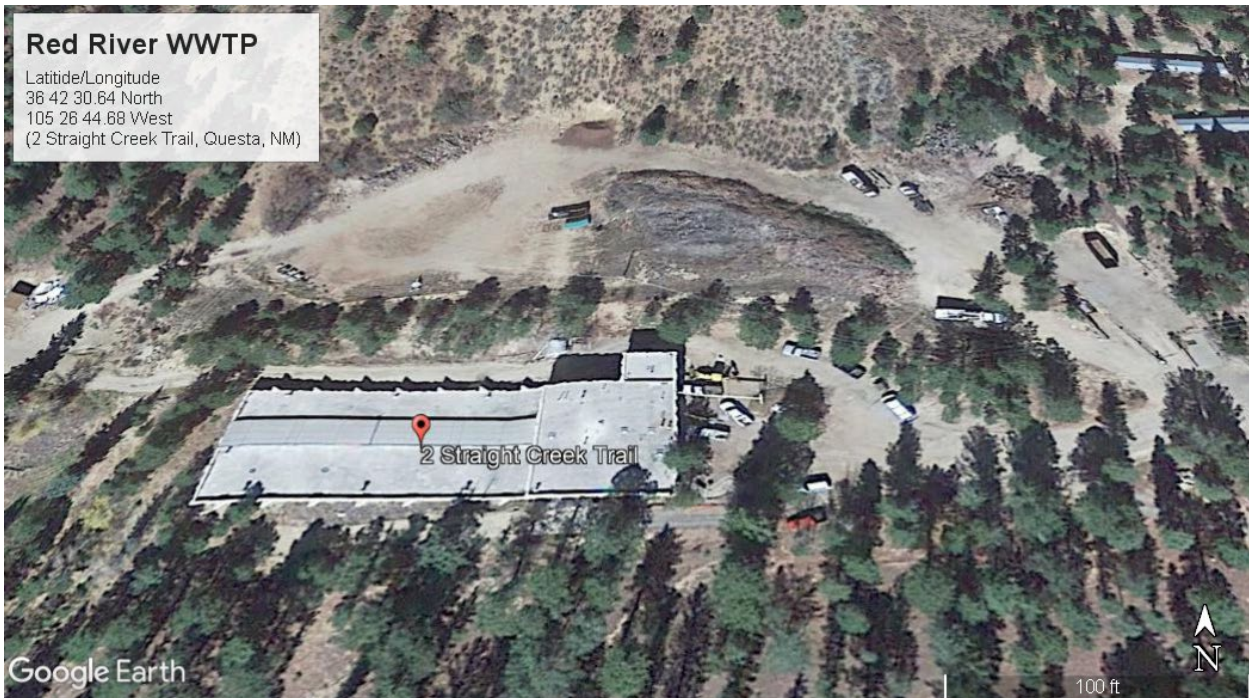
Aerial Image #1: Overall view of the Town of Red River’s Wastewater Treatment Plant. Aerial from Google Earth maps.
