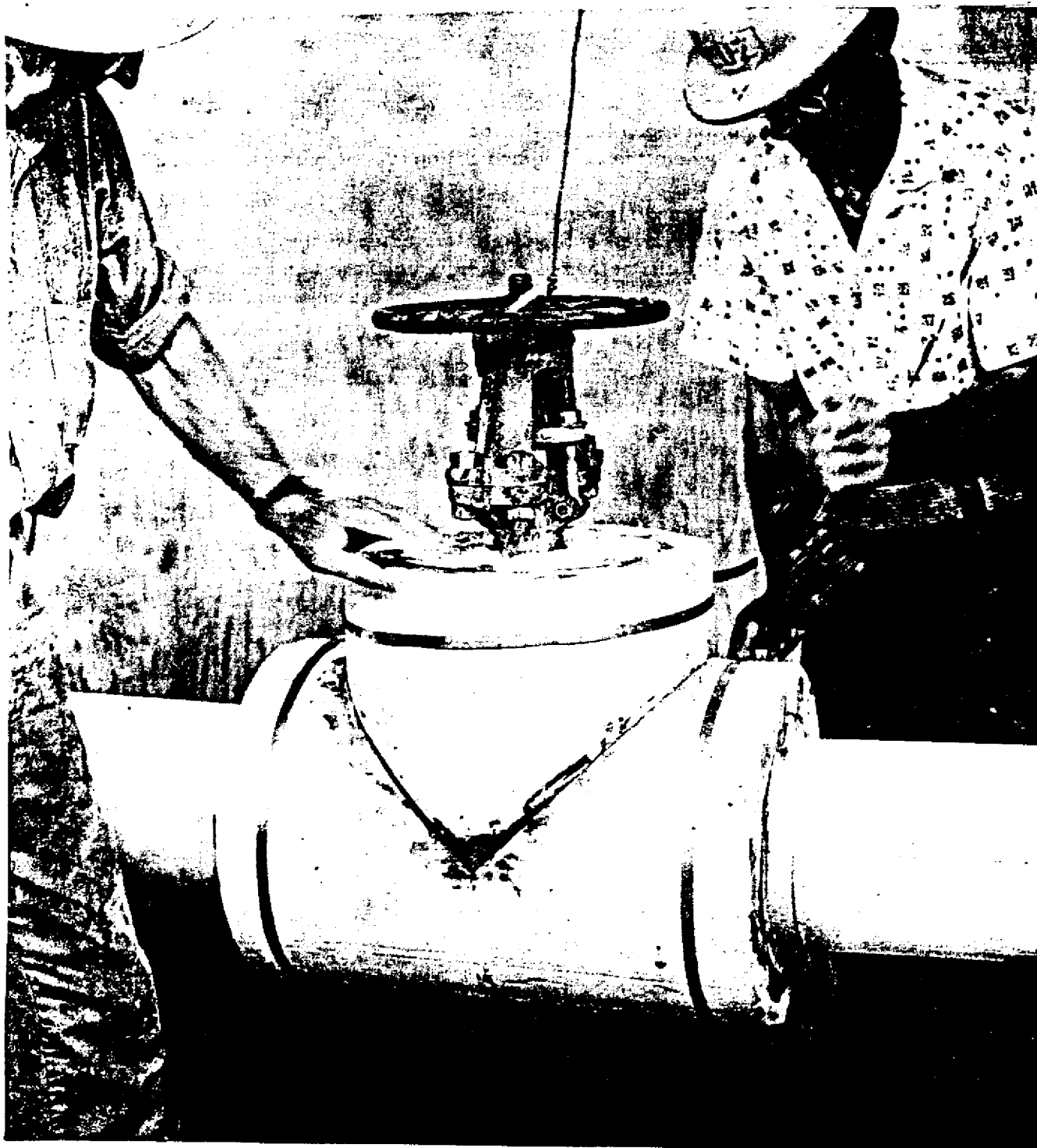
Flanged Globe Valve Cover Secured In Position
