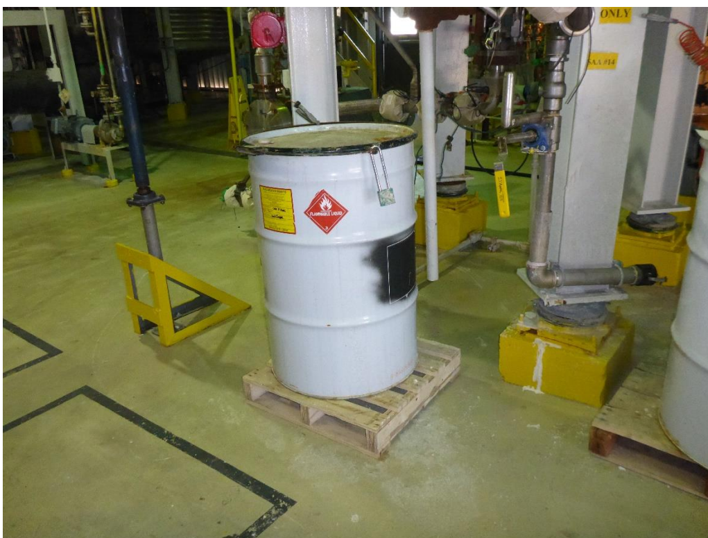
Photo 15: One 55-gallon drum at SAA #13, which is used to accumulate hazardous waste OAA filters that are generated by the OAA process. The drum was labeled hazardous waste OAA filters and identified with a flammable liquid DOT hazard placard.
