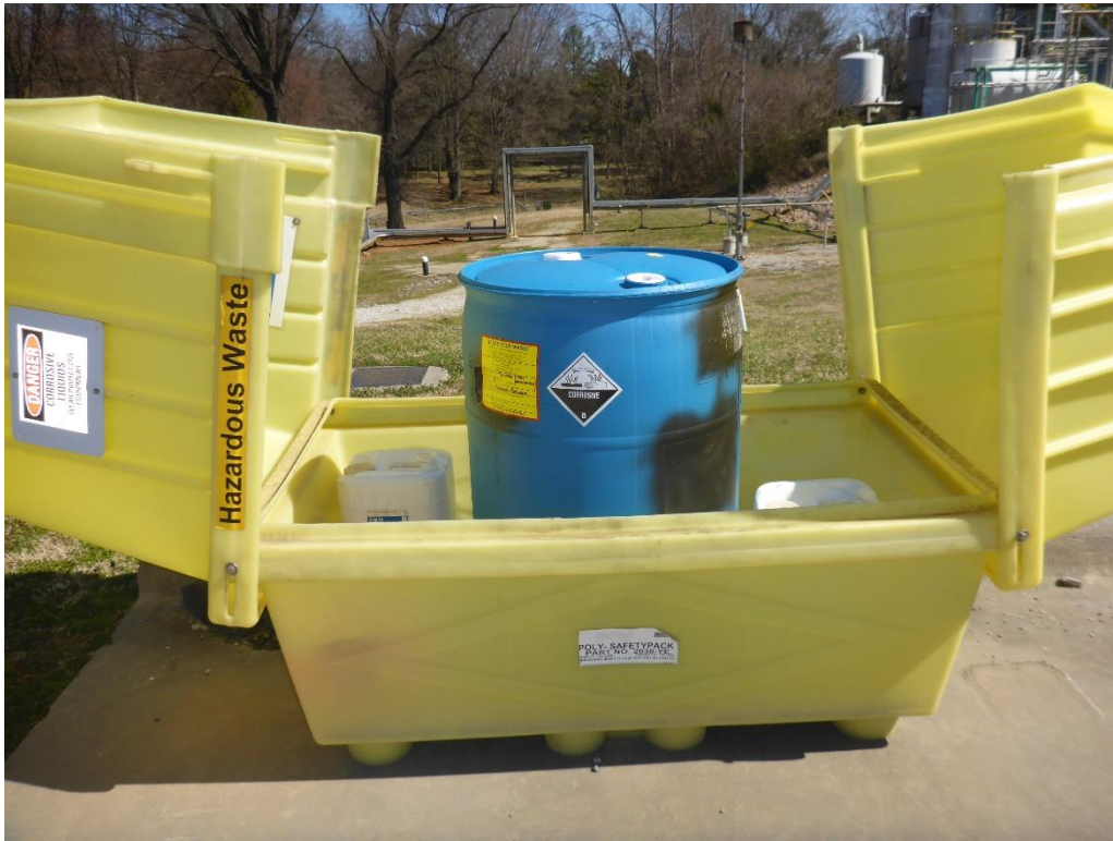
Photo 8: One 55-gallon drum inside a locked, plastic clam-shell secondary containment unit at SAA #7, which is used to accumulate hazardous waste MEA waste that is generated by the MEA flare. The clam-shell was labeled as SAA #7 and “danger corrosive liquids.” The drum was labeled hazardous waste MEA waste and identified with a corrosive DOT hazard placard.
