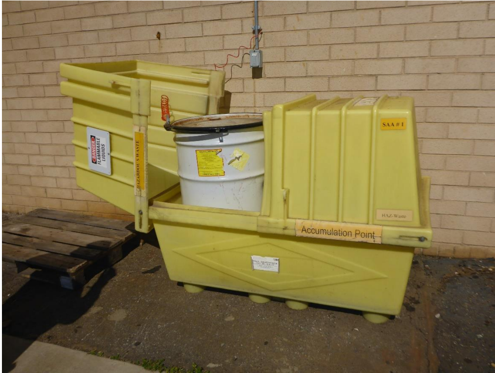
Photo 1: One 55-gallon drum inside a locked, plastic clam-shell secondary containment unit at SAA #1, which is used to accumulate hazardous waste paint cans generated throughout the facility. The clam-shell was identified as SAA #1, labeled hazardous waste and “danger flammable liquids.” The drum was labeled hazardous waste paint cans and identified with a faded flammable liquid DOT hazard placard.
