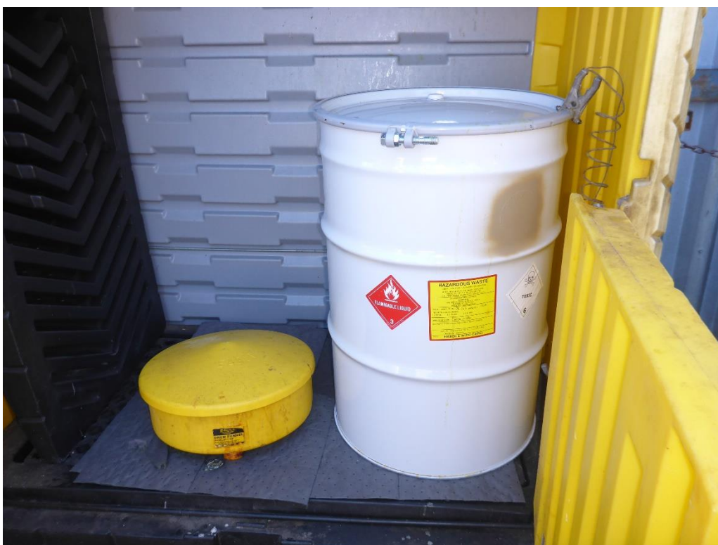
Photo 14: Laboratory CAA between the QC and PD laboratories. The area is a plastic secondary containment shed located just outside the QC laboratory. The area was identified with a sign which read “hazardous waste storage.” Nouryon manages ignitable waste in this CAA, and the shed was also identified with signs reading “danger, no smoking,” and “danger, flammable liquids.”
