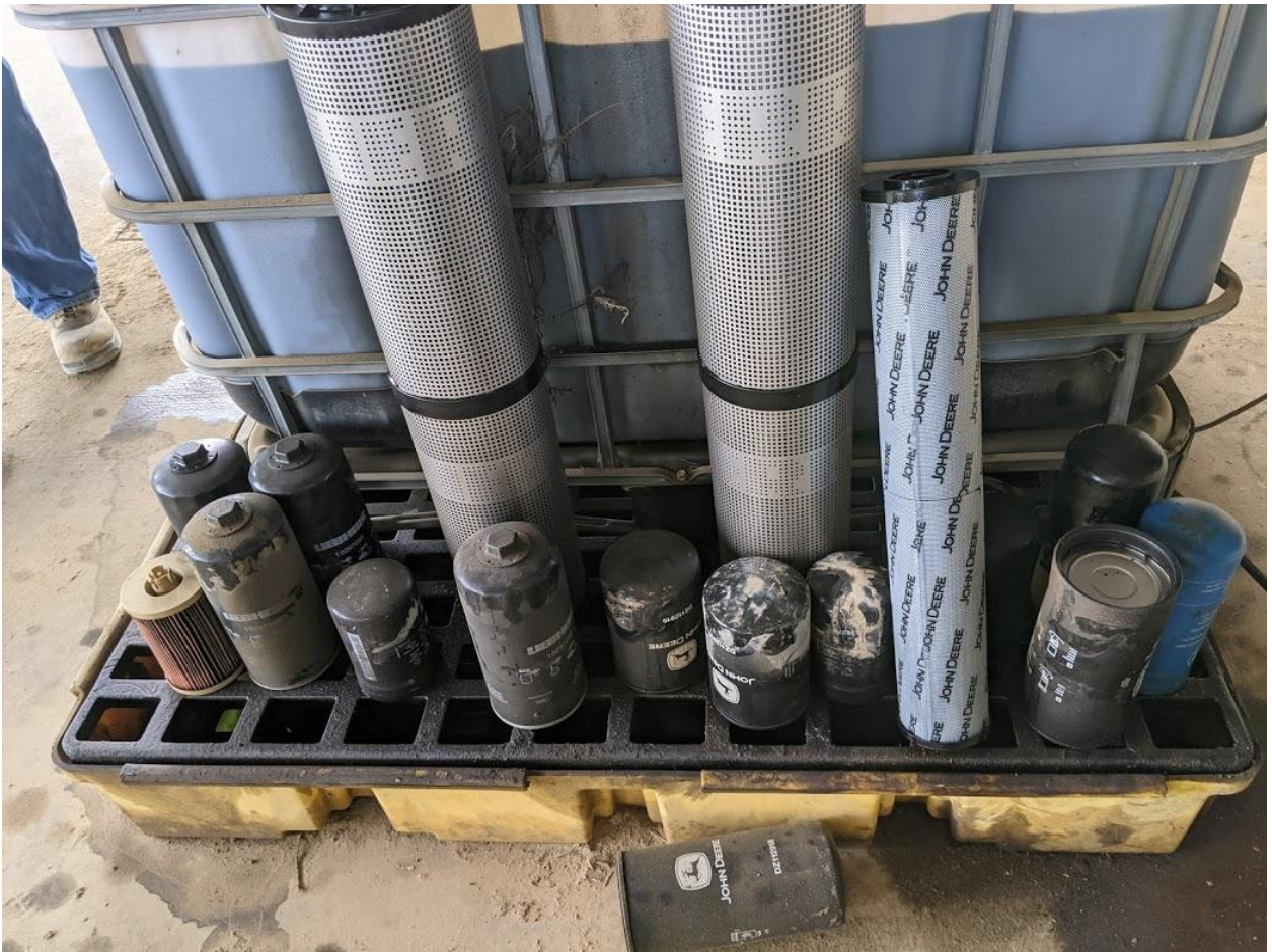
Photograph 3 of 3: Yellow secondary containment for used oil
