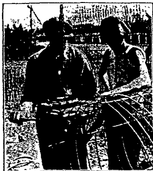
Cables being welded by Allan Portable Welding Machine
