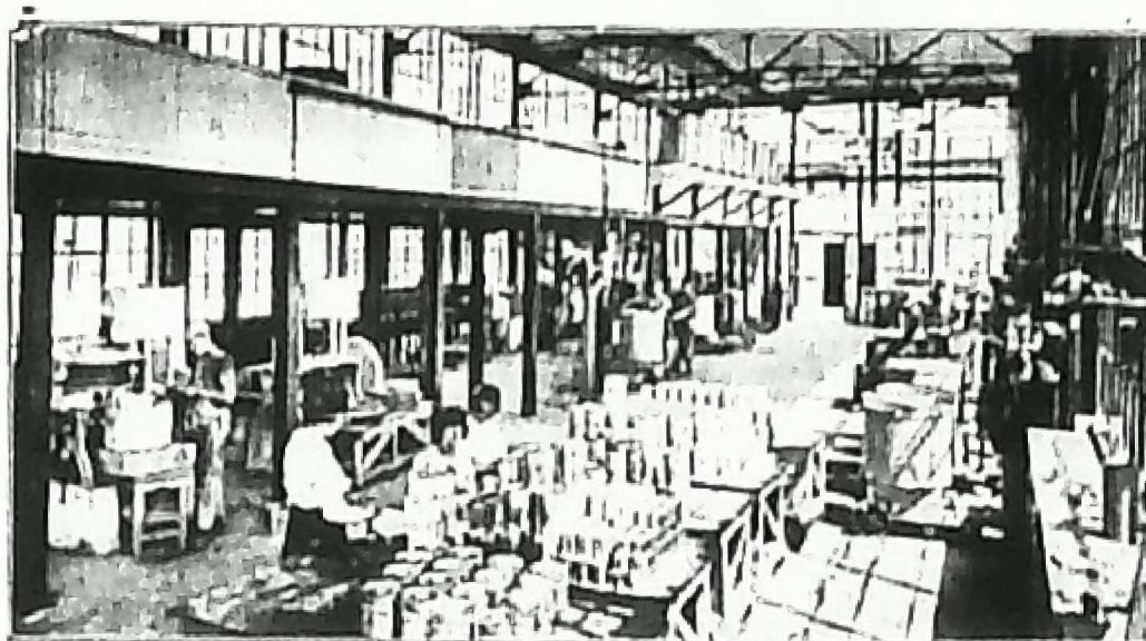
INTERIOR VIEW OF MATHEWS FACTORY UNIT ON SAN FERNANDO ROAD
