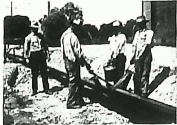
Application of "McEverlast" Electrolysis Proof Coating to 8 inch Gas main of Southern California Gas Company.
