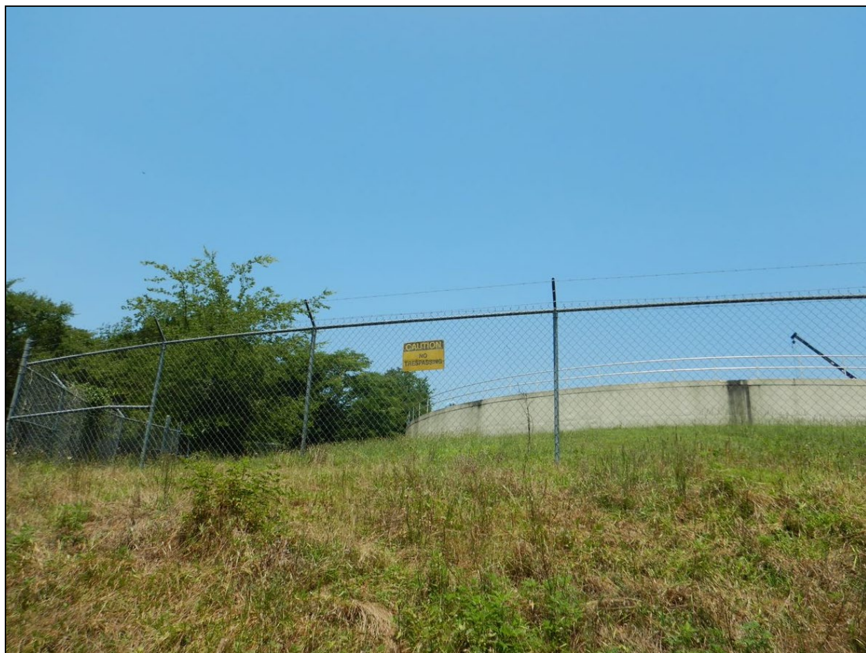
Photograph 2. Perimeter Fence, Ouachita WTP View of the locked barbed wire fence surrounding the Ouachita WTP displaying an additional security sign reading “No Trespassing.”
