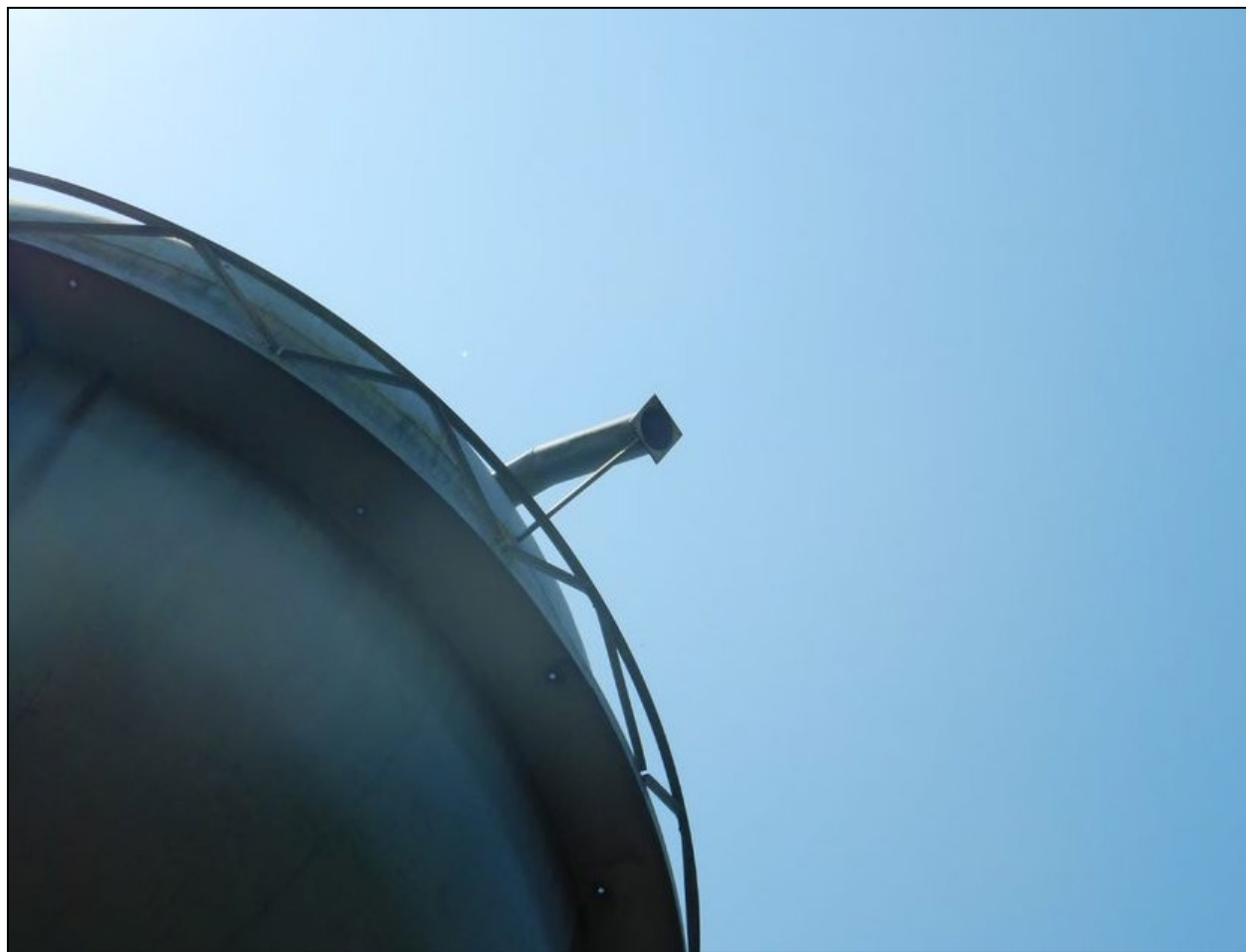
Photograph 5. Backwash Water Storage Tank Close-up view of the overflow pipe extending out of the top of the backwash storage tank. It was unclear if the opening was screened or not.
