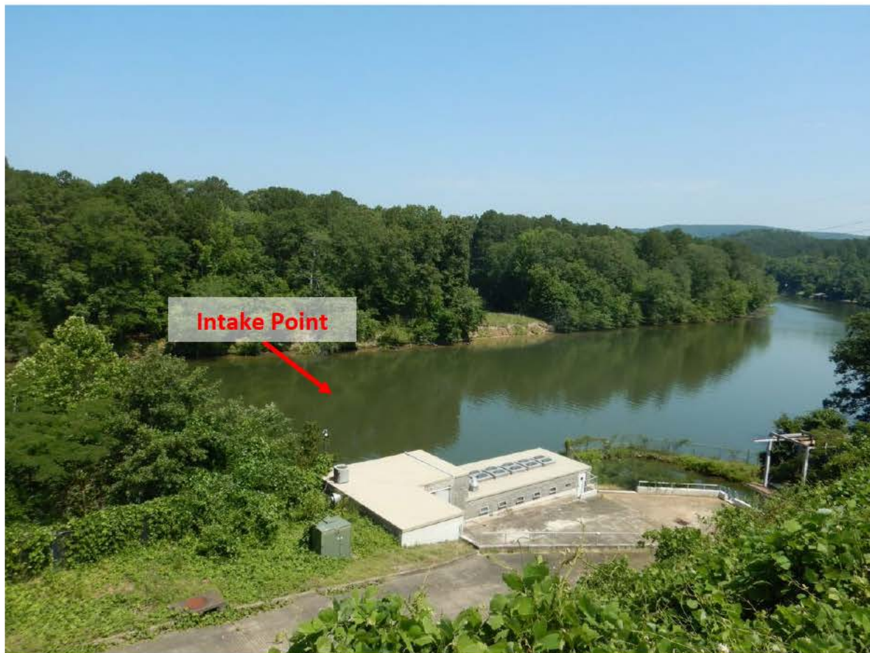
Photograph 3. Raw Water Intake View of the raw water pump station containing five pumps, as well as the raw water intake point in the Ouachita River. There was no buoy representing the intake point, and System representatives stated that the buoy had been washed away during a recent storm.
