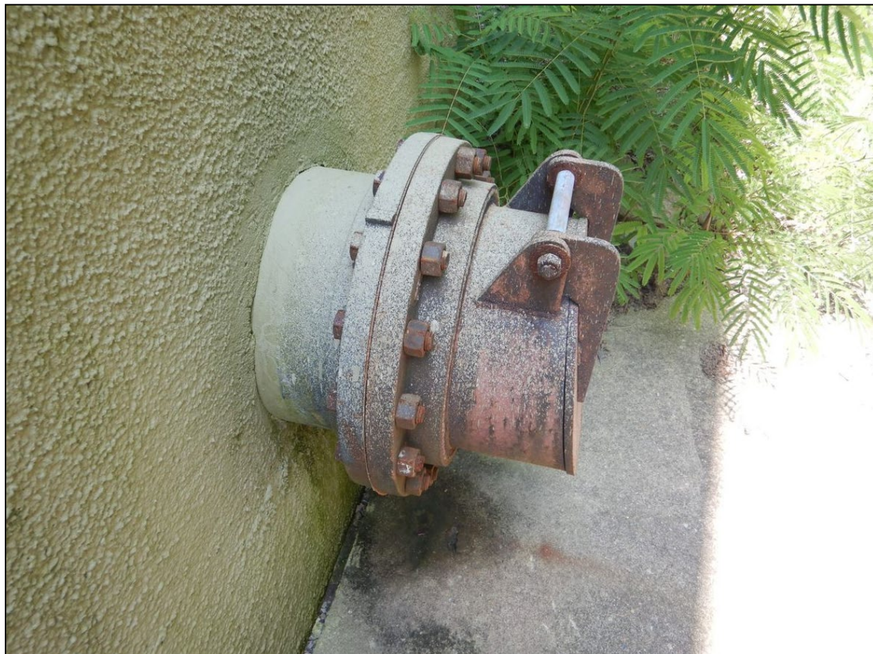
Photograph 44. Overflow Pipe, Music Mountain Water Storage Tank View of the overflow pipe that extended from the tank. The opening was covered by a flapper with a tight seal.
