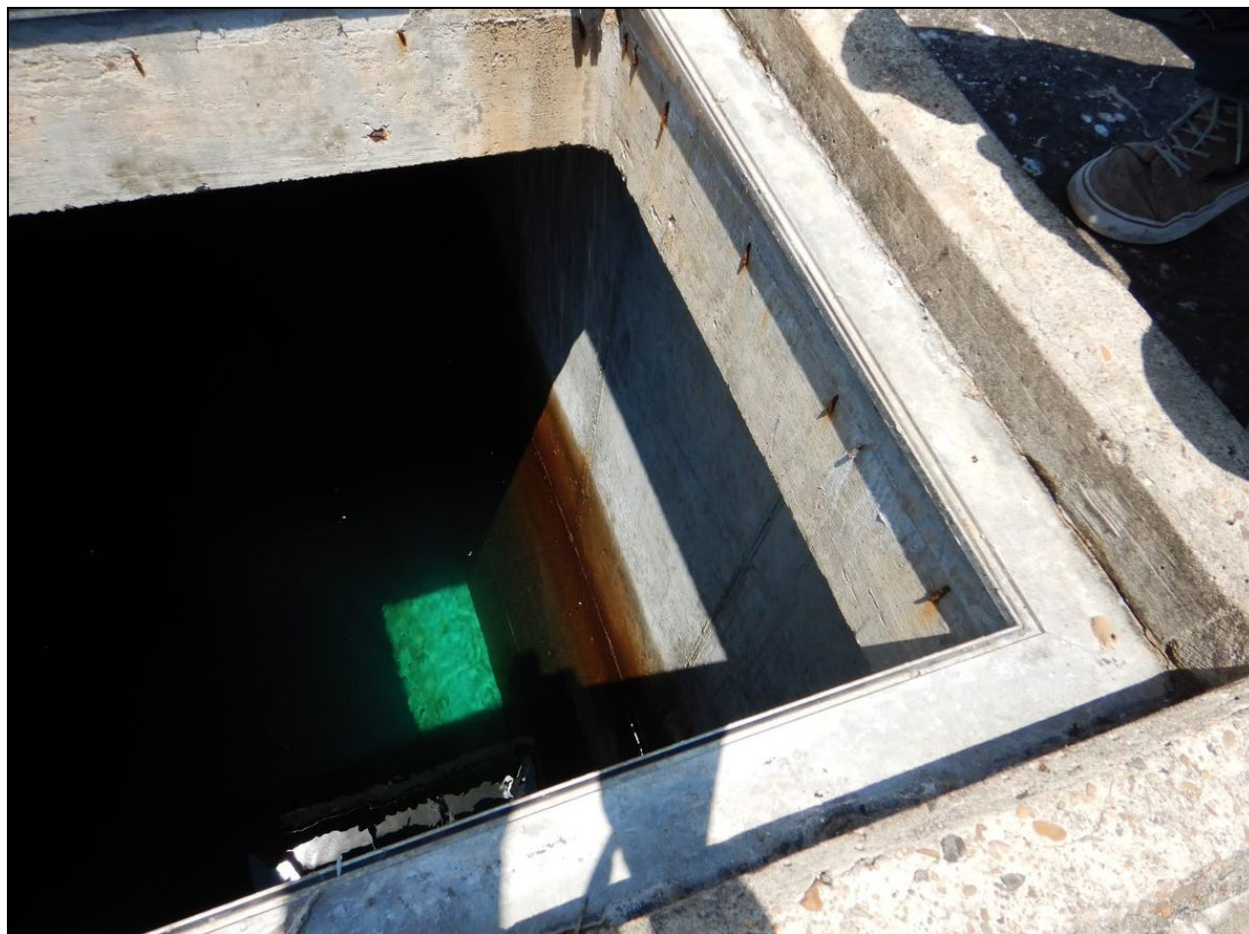
Photograph 30. Hatchway, Clear Well #3 View the inside of the elevated hatchway leading to Clear Well #3. The inside of the hatchway did not contain drainage, and the lid was flush with the top of the tank. If water were to get inside of the lid, it appeared that it would pool over the hatch and possibly get into the clear well.
