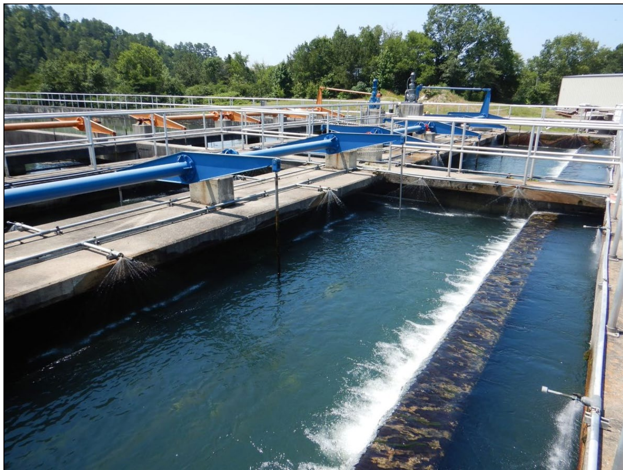
Photograph 20. Flocculation Chamber, Sedimentation Basin No. 6 View of the flocculation chamber associated with Sedimentation Basin No. 6. A slow mix was occurring in the chamber to try to generate floc.
