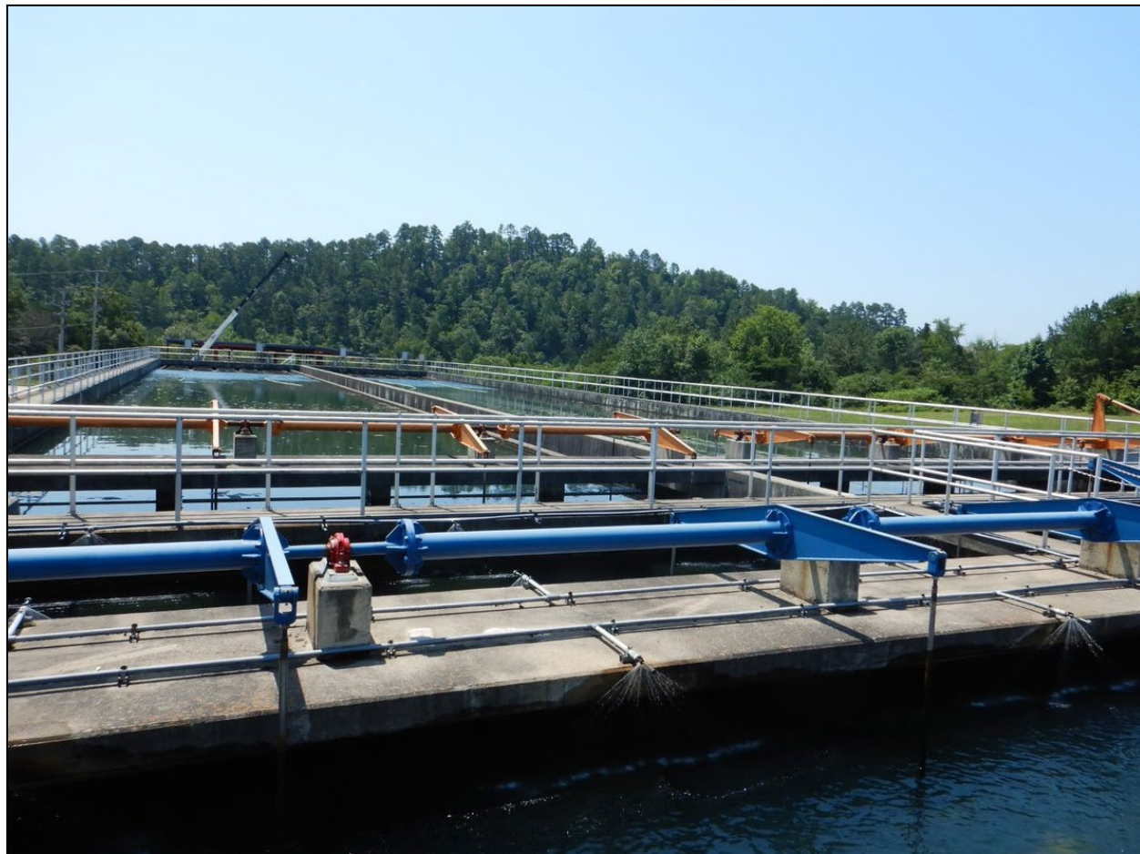
Photograph 19. Sedimentation Basin Nos. 6 and 7, Ouachita WTP View of Sedimentation Basin Nos. 6 and 7, which are clustered in a separate area from Basin Nos. 1-5.
