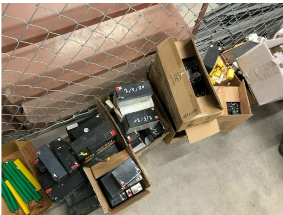
Photo 30 – 13 boxes of universal waste batteries not properly labeled or marked with an accumulation date.
