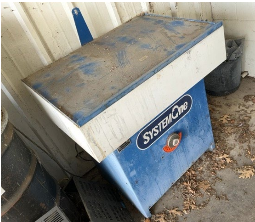
Photo 40 – unused Parts Washer in maintenance shop that contained liquid sat the time of the inspection.
