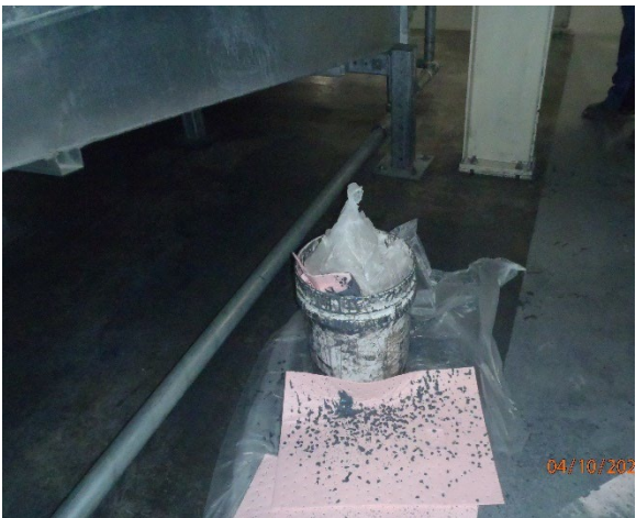
Picture 8 – Primer Purge Recovery System clean up debris
