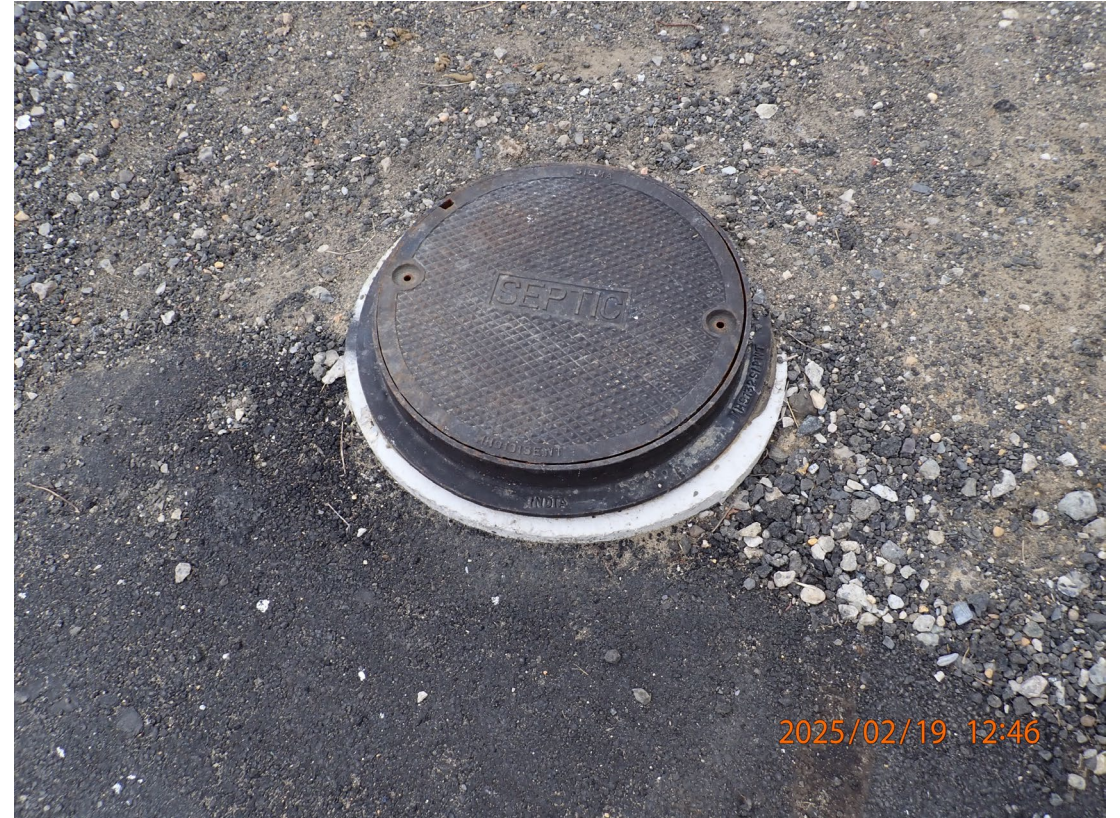
P2190040 – Septic tank cover.
