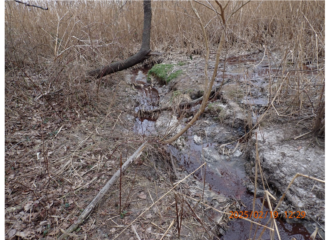
P2190032 – Red, unauthorized discharge leaving the southeastern portion of the spray field.
