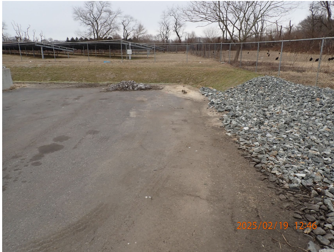
P2190041 – Retention pond on the eastern portion of the Site.
