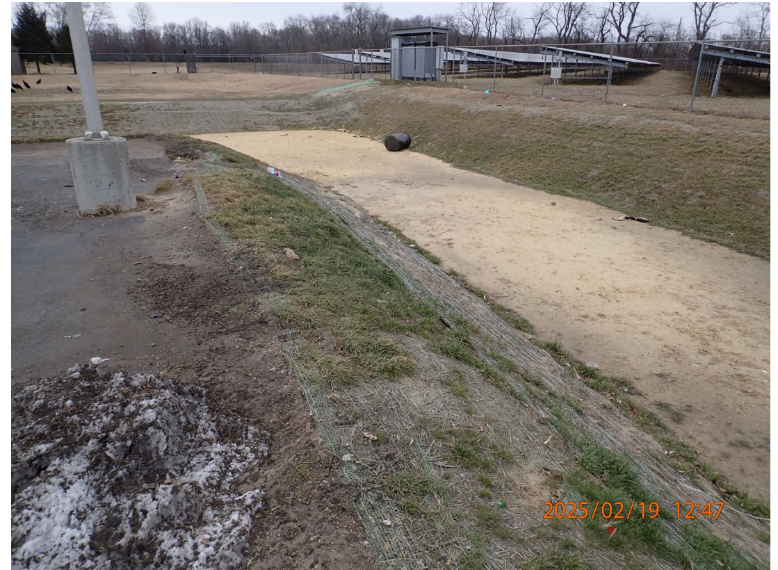
P2190042 – Retention pond on the eastern portion of the Site.
