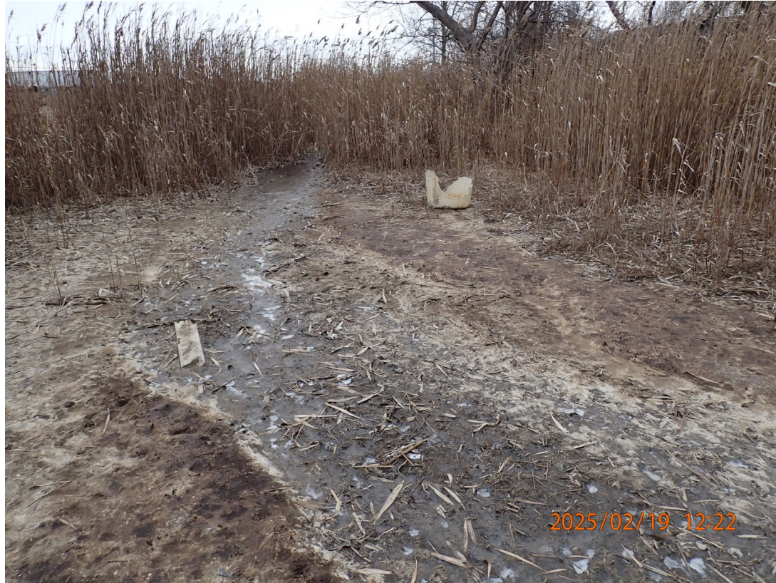
P2190025 – Erosion in the southeastern portion of the Site.
