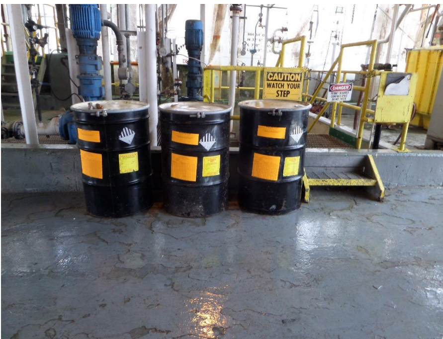
Photograph 4: Three 55-gallon Hazardous Waste Drums in Central Accumulation Area
