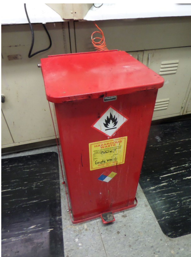
Photograph 6: SAA Container with HW Label and Hazard Marking
