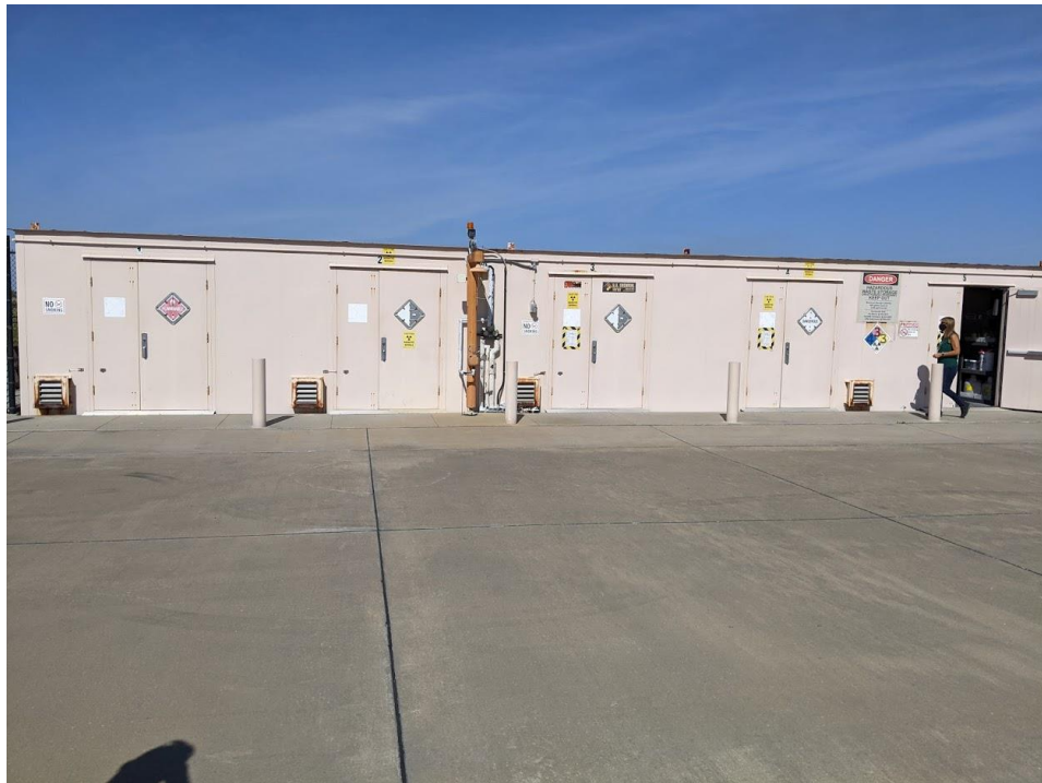
Photograph 3 of 4: Locker Storage
