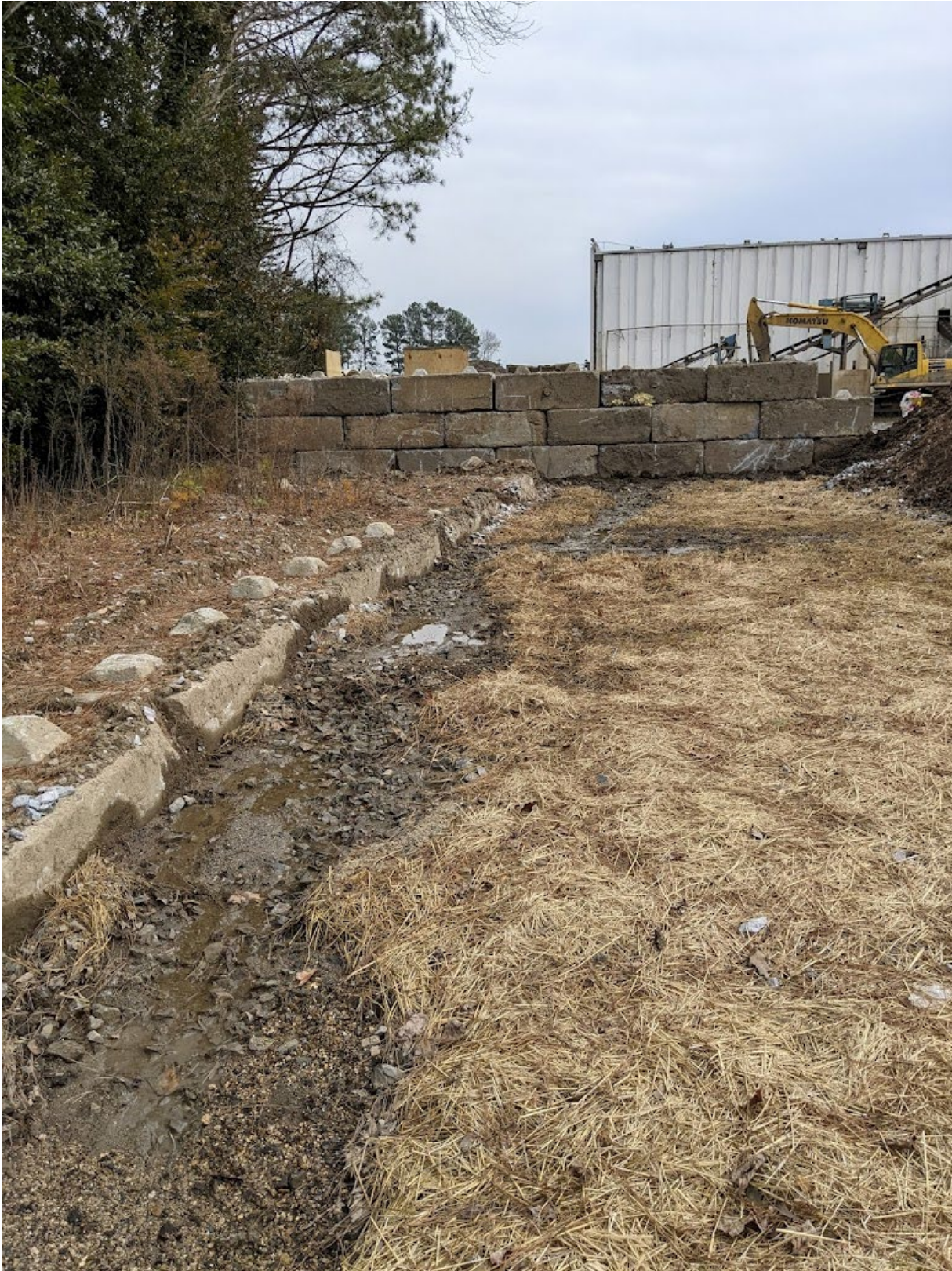
Photograph 18 of 30: Back Side of Unfinished Wall in Jig Pad Area that Leads to Outfall 003
