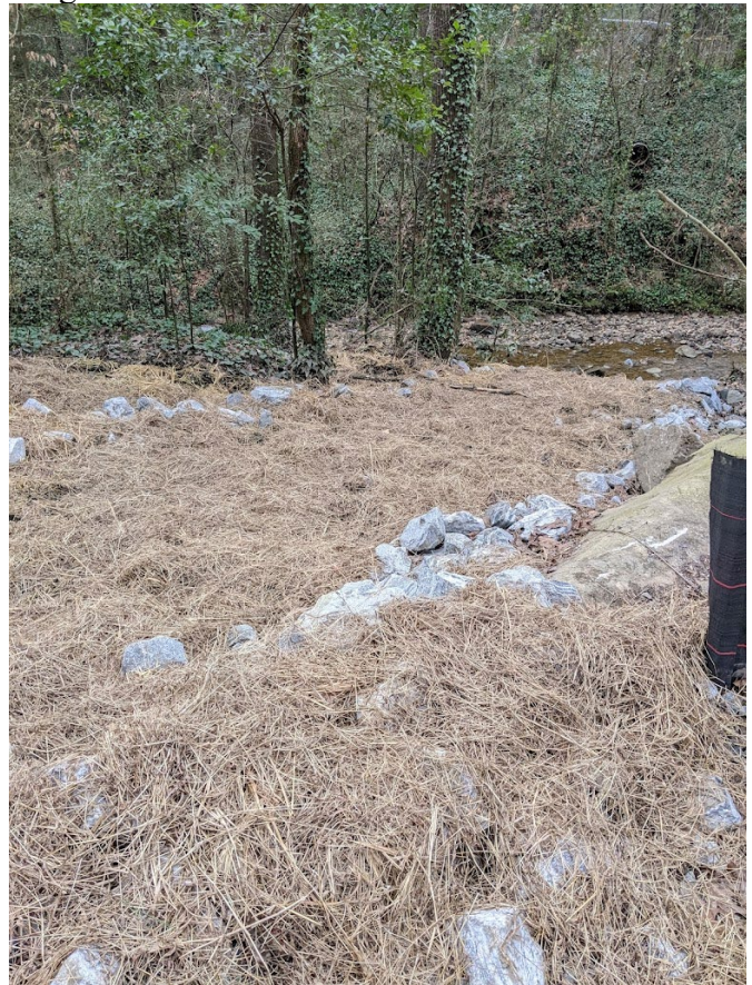
Photograph 24 of 30: Outfall 002 with Riprap
