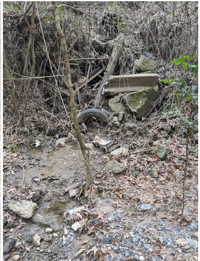
Photograph 26 of 30: Outfall from Storm Drain in Photograph 11
