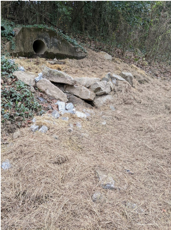
Photograph 23 of 30: Outfall 002 with Riprap
