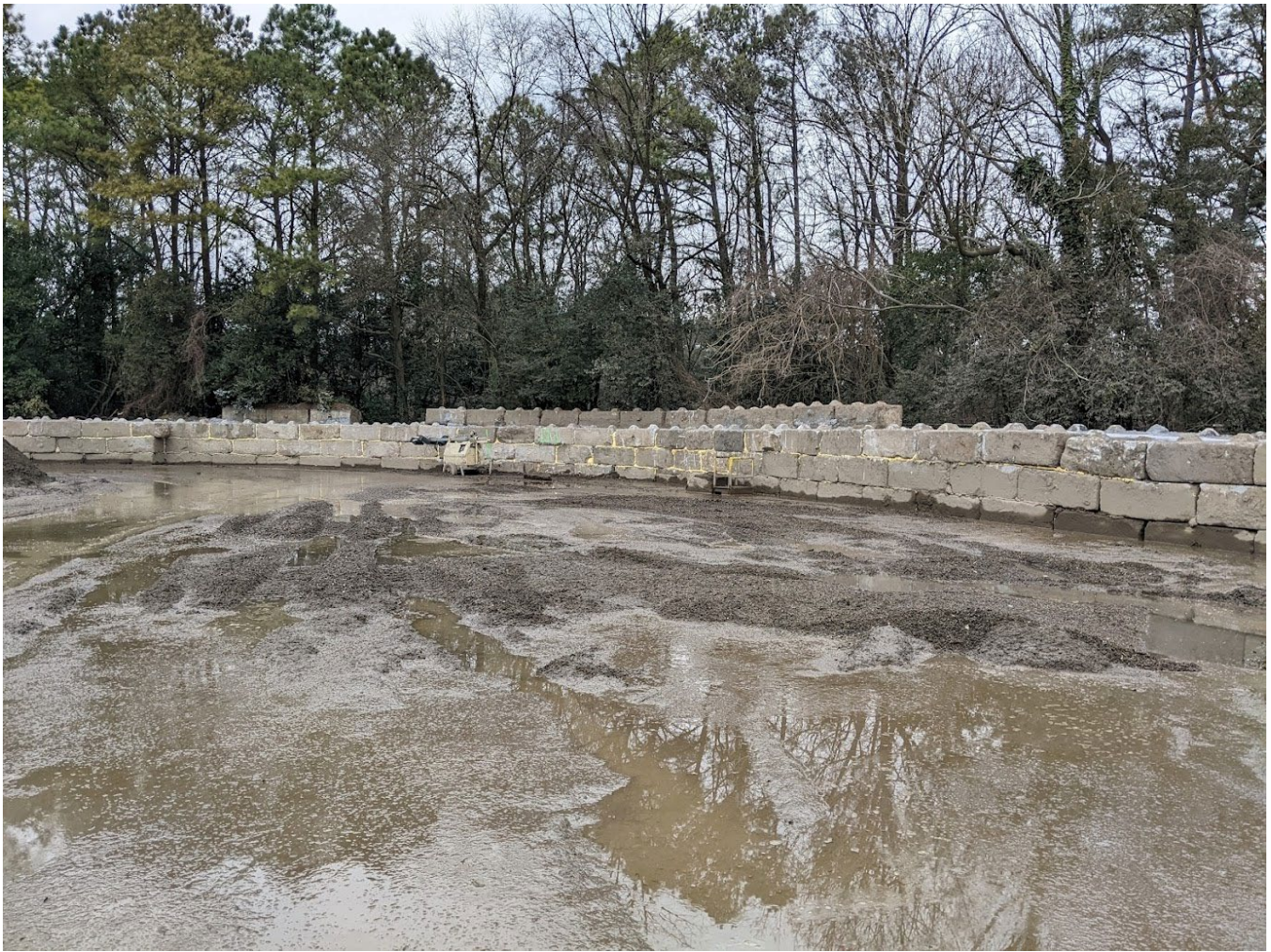
Photograph 8 of 30: Jig Pad Area Wall Addition
