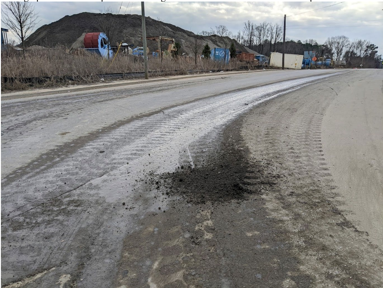
Photograph 2 of 30: Material Spillage onto Empire Blvd. off the Back of the Dump Truck
