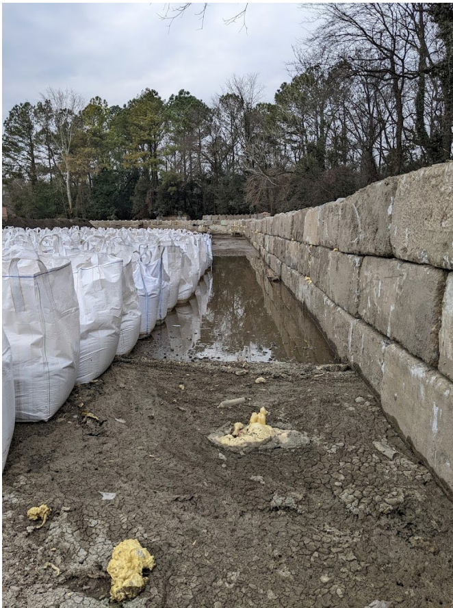
Photograph 6 of 30: Jig Pad Area Wall Addition
