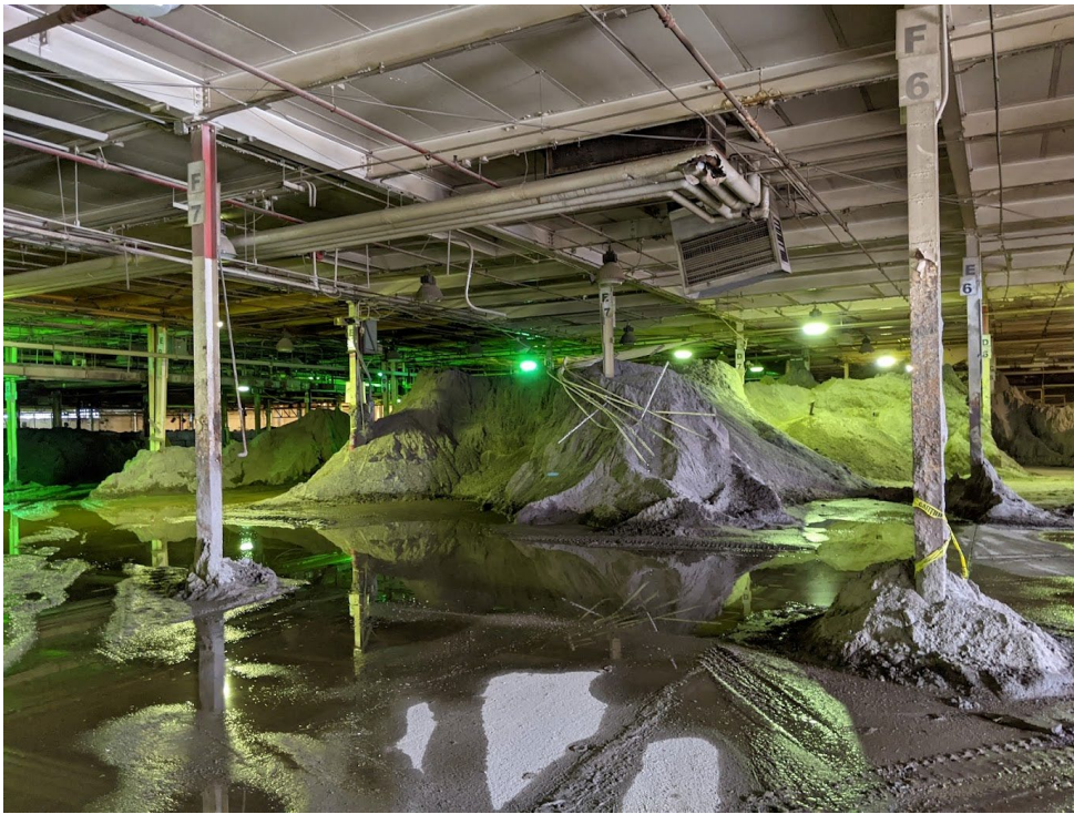
Photograph 22 of 30: Material Stored in Keebler Building
