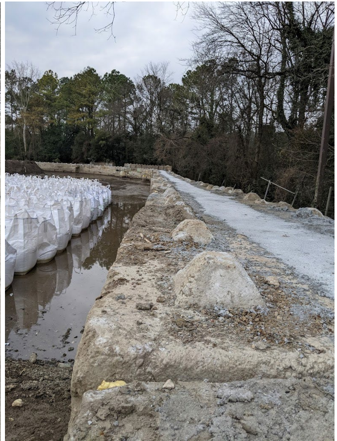
Photograph 7 of 30: Jig Pad Area Wall Addition
