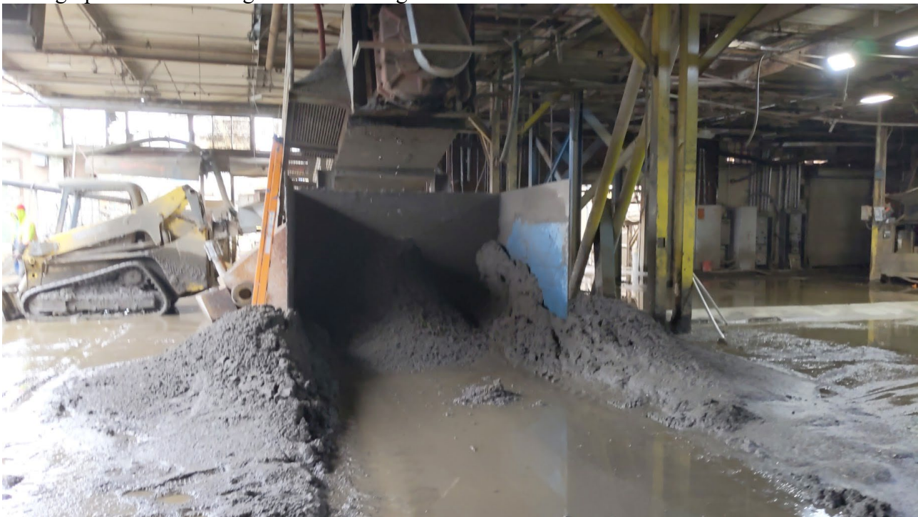
Photograph 20 of 30: Sludge from Screw Process Stored on the Ground in the Process Area
