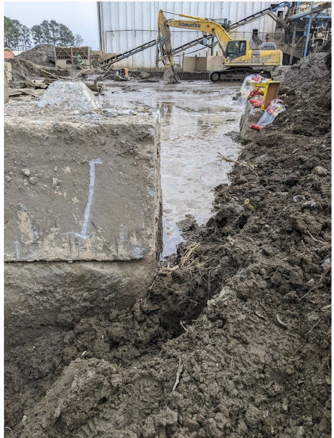
Photograph 16 of 30: Unfinished Wall in Jig Pad Area
