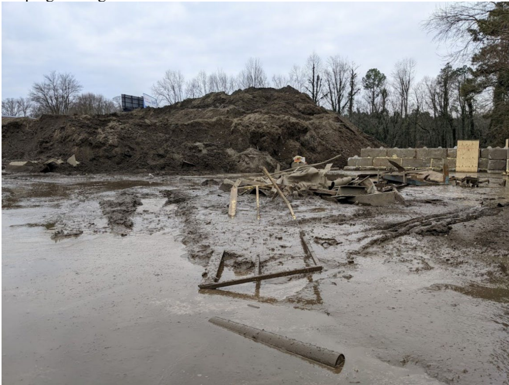
Photograph 17 of 30: Unfinished Wall in Jig Pad Area
