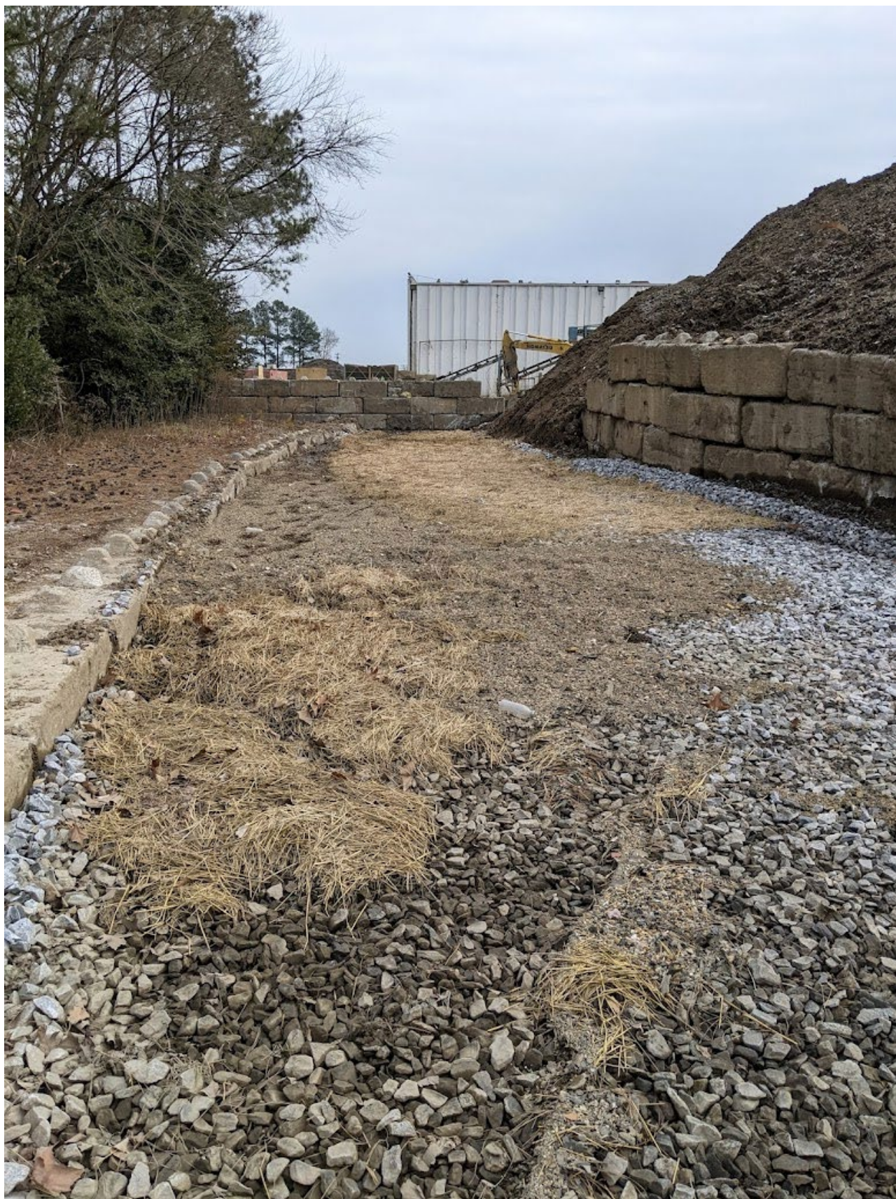
Photograph 9 of 30: Backside of Unfinished Wall in Jig Pad Area that Leads to Outfall 003
