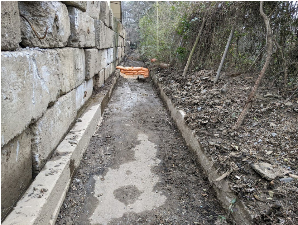
Photograph 10 of 30: Storm Drain Behind Jig Pad Area Wall
