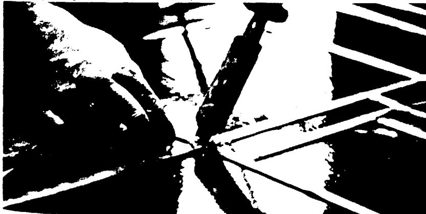
Technique by which glass panes are "lead" into place.
