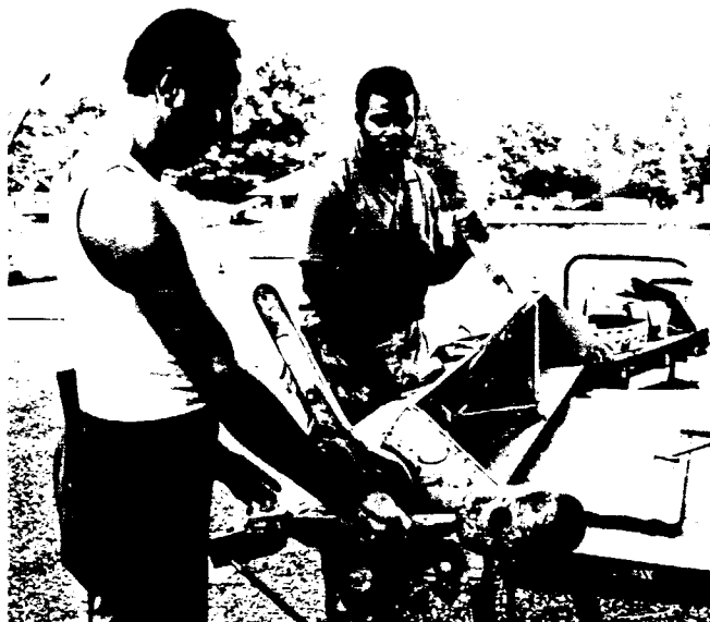
Workmen put the first fold in the lead at the sheet metal "shop" assembled on the roof by the roofing contractor.
