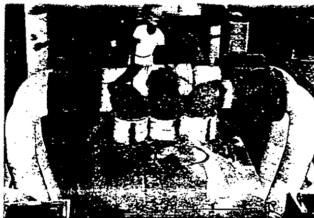
Kaylo-20 Pipe Insulation is adaptable to vessels of unconventional size and shape. Used on pipes, breechings, ducts and boilers, it is shown here on steam lines of a power station's turbines.
