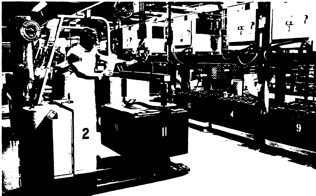
The battery/truck/maintenance/charging area at R. T. French's Souderton, Pa. facility includes an overhead hoist for safe removal of batteries for charging from the company's electric lift truck fleet.
