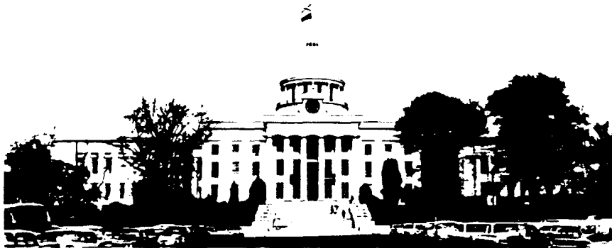
Alabama's State Capitol in Montgomery is one of the most impressive in the country. Much of the terne-coated steel on dome, promenade and supporting drum remains in excellent condition today, 128 years after its installation.
