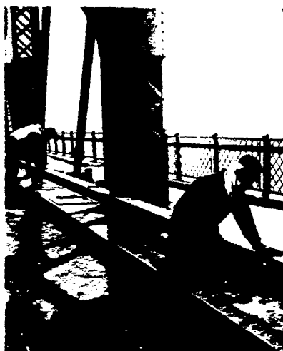
Workmen remove old paint and rust prior to application of anticorrosive lead paint.
