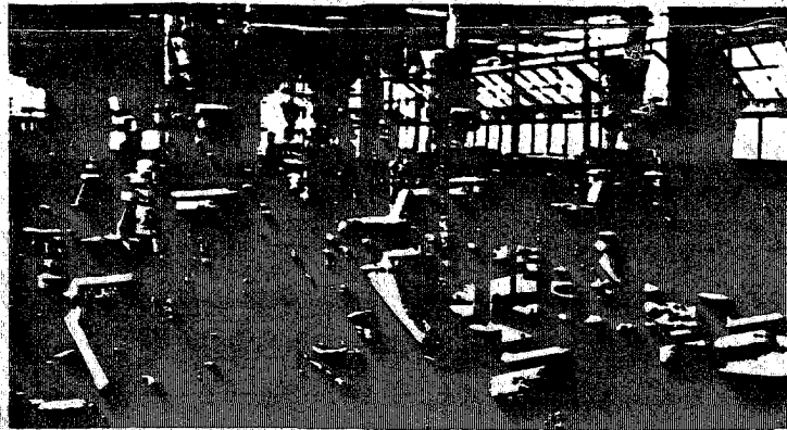
1921 . . NEW ENAMEL DEPARTMENT added to provide for much increased demand for high quality enamels and other liquid paints. Equipment fifteen tandem mills, four roller mills, thirty-eight mixers, thirty-eight thinning tanks. Daily capacity 4,000 gallons.
