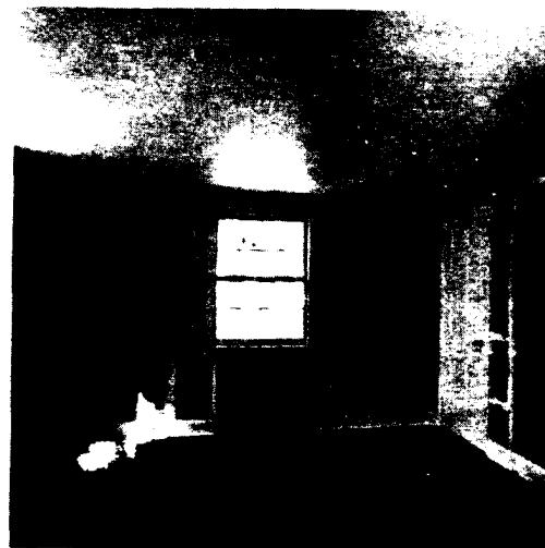
A bedroom in this small home. The plywood ceiling has been painted three coats of white lead, as well as trim, and the joints in the walls finished smooth for the wall decoration
