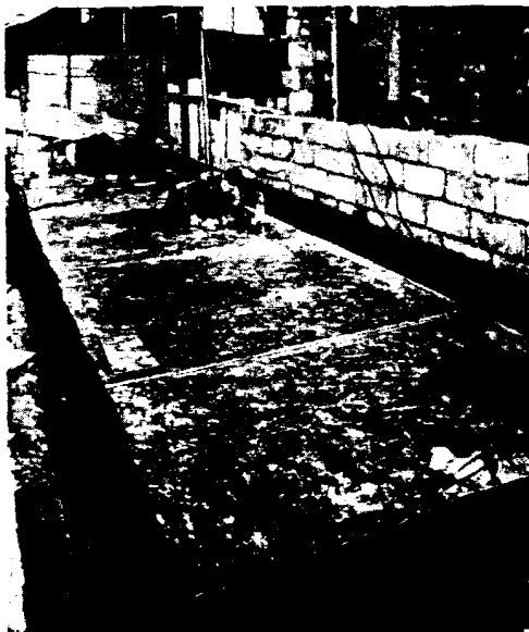
Fabricating the large 8-lb. sheet lead pan under the soda-fountain of Liggett's Drug Store in Grand Central Terminal, New York
