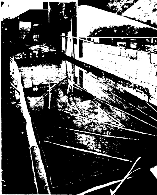
The completed sheet lead pan for the Liggett's Drug Store fountain, with all its bleeders installed and the sleeves wiped to the water pipes. The pan has been filled with water for a 24-hour test
