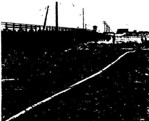
Close-up of the Atlantic City service attached to the cable and placed on rollers
