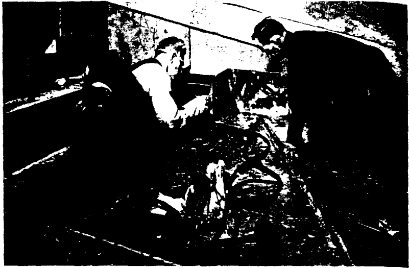
Burning a vertical corner joint. All seams in the pans were lead-burned. Note, also, the bleeder with the V notches leading from the corner
