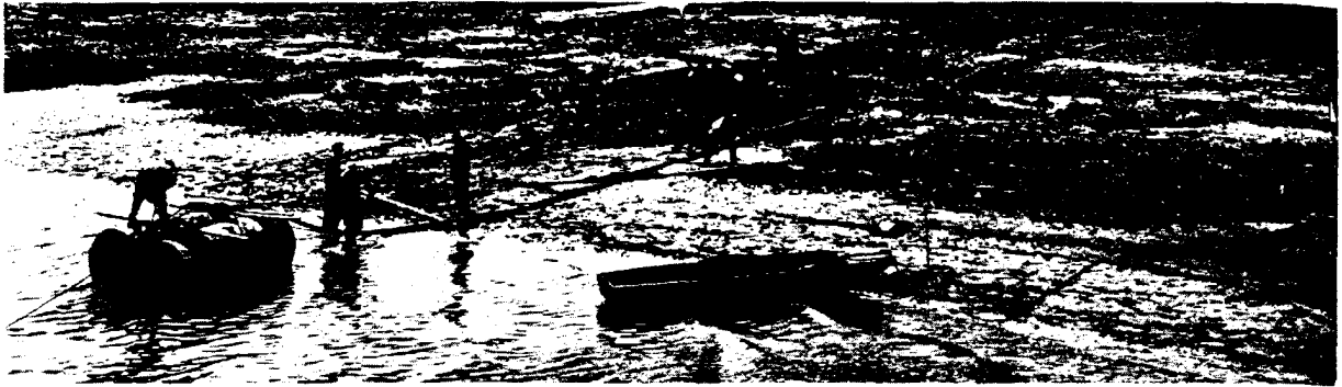
View showing a float with 2-in. lead service attached ready to be drawn across a waterway in Atlantic City, New Jersey
