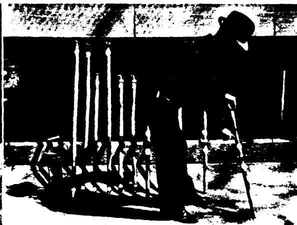
At left, the new lead service, replacing the one which failed, wiped to the curb stop and to the meter connection. At right, a Chicago Water Dept. foreman points out the Seal of Approval on a group of lead services
