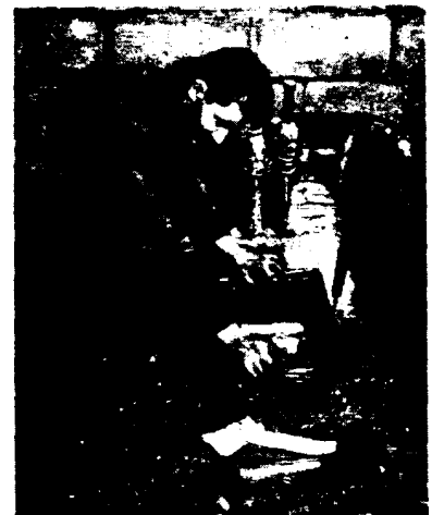
Preparing the joint between one of the three sump linings and the main pan
