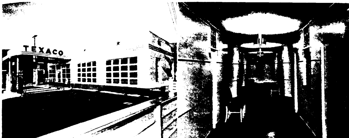
Left, a new Texaco Service Station at Tacoma, Washington, designed by the Texaco staff architects using plywood painted with white lead for the exterior. At right, interior plywood decorated with white lead for the Andrews Apparel Shop, also in Tacoma. Russell, Lance and Muri, Tacoma, were the architects
