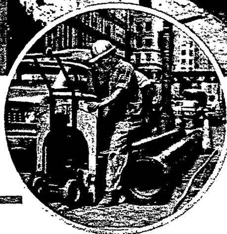
CLOW Ductile Cast Iron Pipe can be cut to length on the job.
