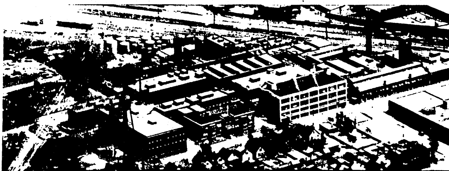
Aerial View of Plant Showing General Layout and Type of Construction. Storage Tanks in Rear.
