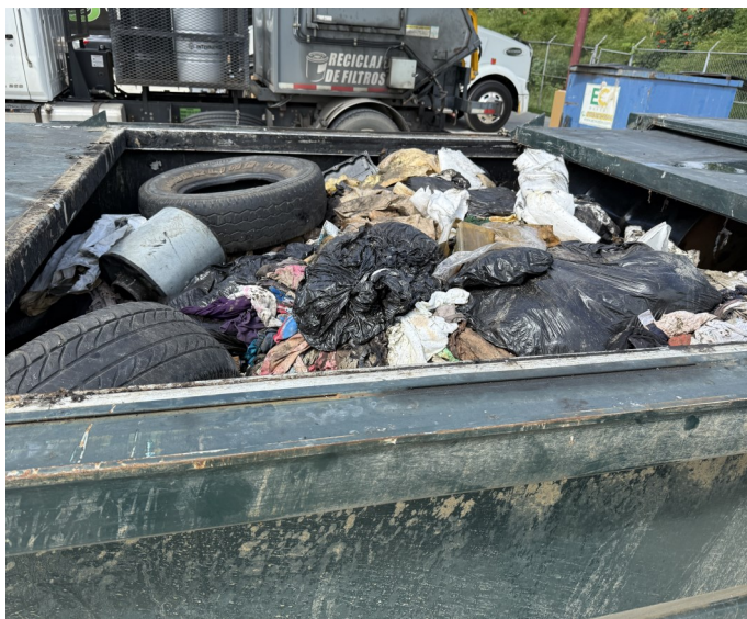
Picture 27-OIL ENERGY SYSTEMS- At the Backyard Dumpster Area there was one (1) 20-yd 3 with oily impacted rags, absorbent pads used oil and fuel oil at the at the generator facility was not labeled or marked clearly with the words “Used Oil,” nor hazardous waste determination of the contents of the container.
