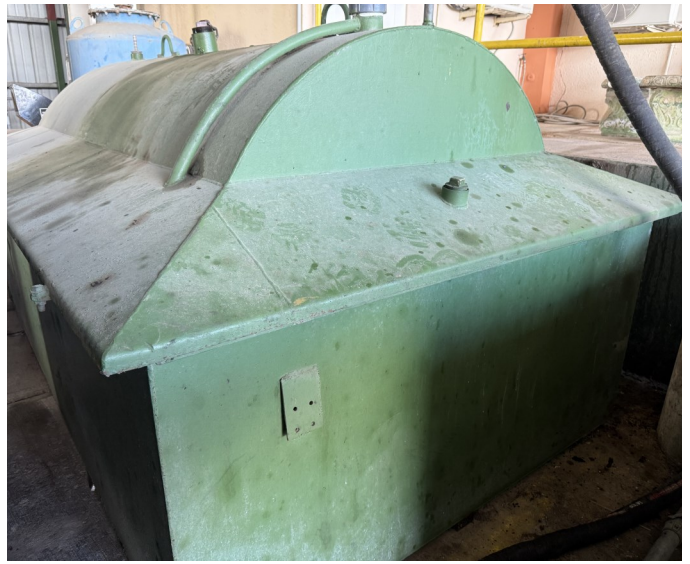
Picture 6 - OIL ENERGY SYSTEMS- At the Used Oil Filters Processing Area there was one (1) 1,000-gallon double steel tank with used oil not labeled or marked clearly with the words, “Used Oil.”
