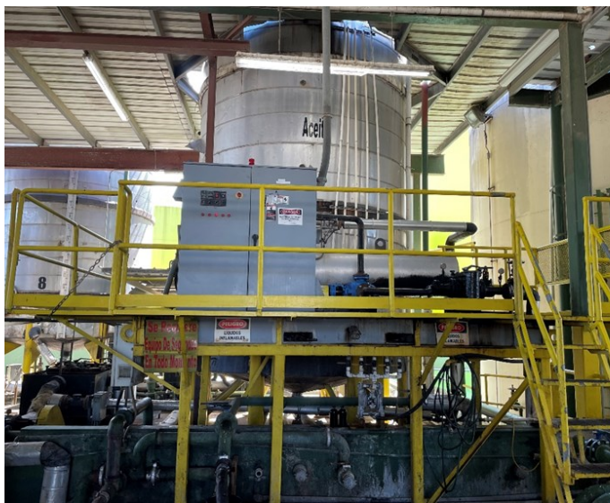
Picture 15-OIL ENERGY SYSTEMS- At the Tank #6 Decanting Process Area there was one (1) aboveground Tank #6 with storage capacity of 17,571-gallons used to store and process used oil at the generator facility was not labeled or marked clearly with the words “Used Oil,.”
