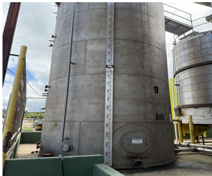
Picture 23-OIL ENERGY SYSTEMS- At the Tank #9 Decanting Process Storage Area there was one (1) aboveground Tank #9 with storage capacity of 30,226-gallons used to store and process used oil at the generator facility were not labeled or marked clearly with the words “Used Oil.”
