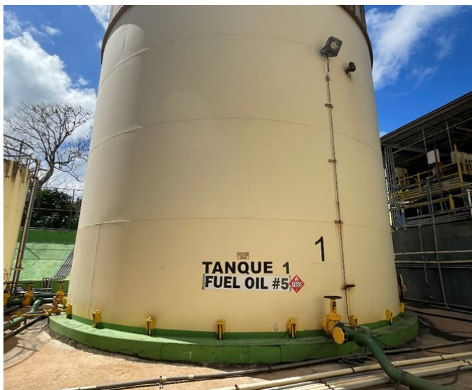
Picture 19-OIL ENERGY SYSTEMS- At the Tank #1 Decanting Fuel Oils Storage Area there was one (1) aboveground Tank #1 with storage capacity of 422,382-gallons used to store fuel oils mixed with used oil at the generator facility was not labeled or marked clearly with the words “Used Oil.”
