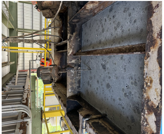
Picture 8 - OIL ENERGY SYSTEMS— At the Wastewater Treatment Plant there were (3) three settling clarifiers where 99% of the suspended solids are separated with contact water and oils emitting strong odors of hydrocarbons.
