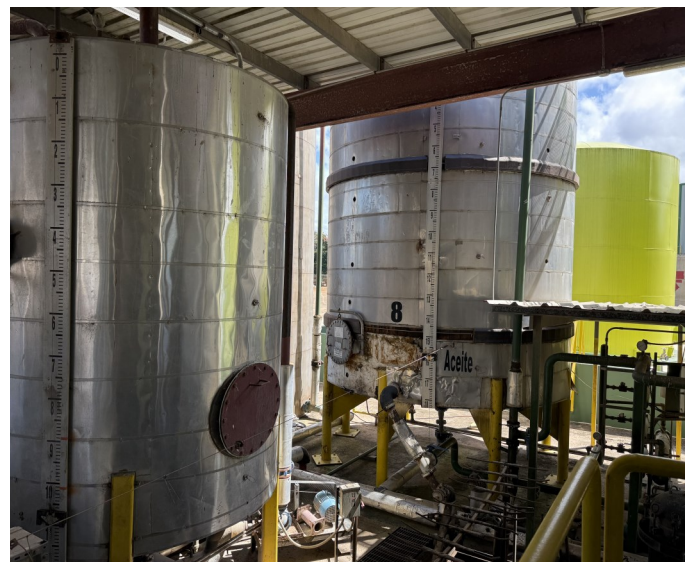
Picture 16 - OIL ENERGY SYSTEMS- At the Tank #7 and Tank #8 Decanting Process Area there were two (2) aboveground Tank #7 and Tank #8 both with storage capacity of 21,302-gallons used to store and process used oil at the generator facility were not labeled or marked clearly with the words “Used Oil,.”
