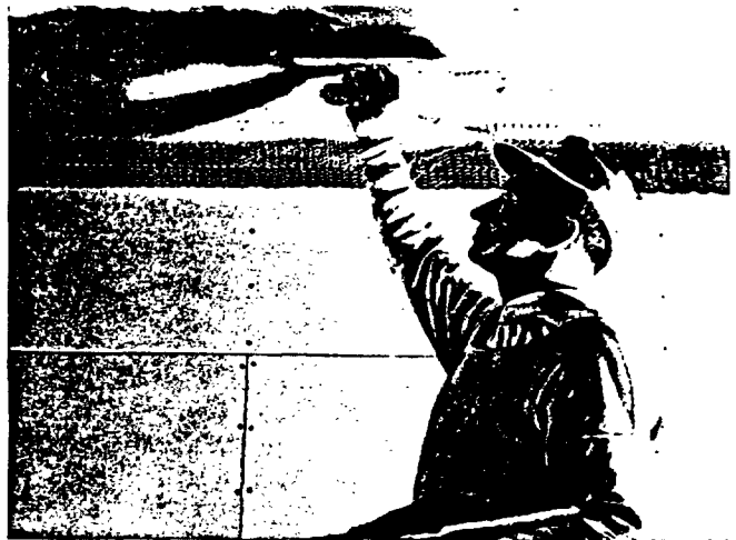
Uniform suction of Rocklath prevents plaster from slipping during application.
