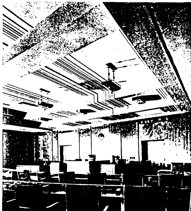
Acoustone ceiling, County Court House, Oshkosh, Wis. Architect: Granger and Bollenbacher, Chicago, Ill.
