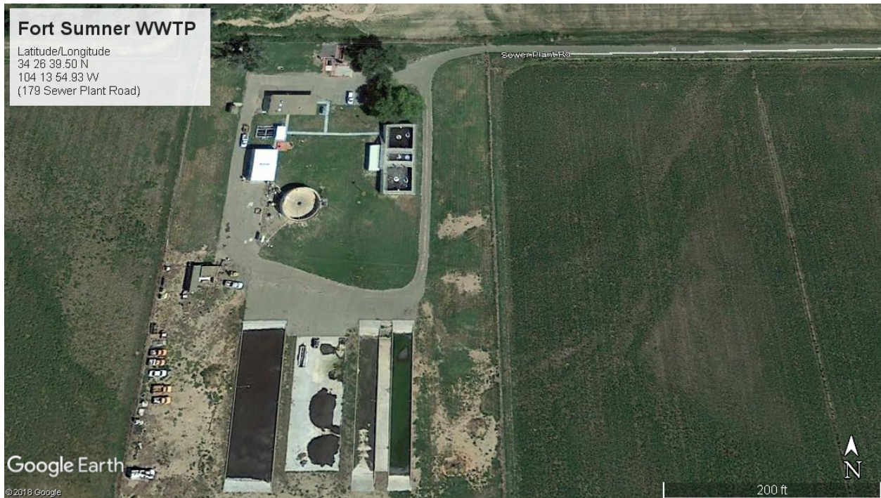
Aerial #1: Overall view of the Village of Fort Sumner Wastewater Treatment Plant. Aerial from Google Earth maps.
