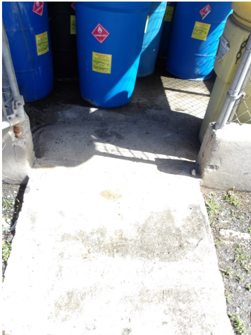
Picture 100-028 Ramp Access for HWSA
