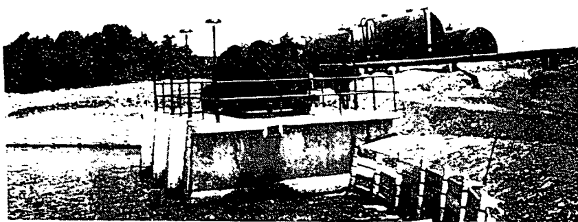
CIRCULATING-WATER INTAKE draws water from Ashe's River bottom to assure ample cooling supply. Day tank, condensate drain tank (starting oil tank (in back)
