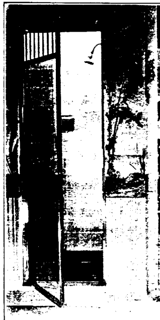
COURTESY DOMESTIC ENGINEERING Lead waterproofed shower room installed on this job.
