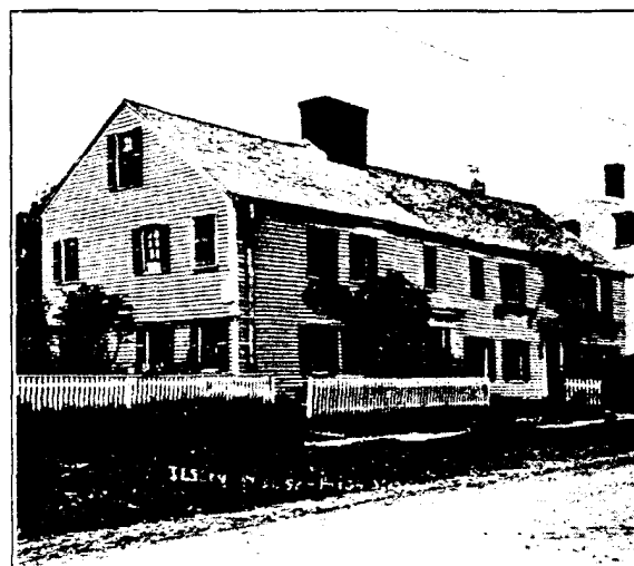
This house, built in 1670, is in excellent condition, thanks to the great protection of lead paints.
