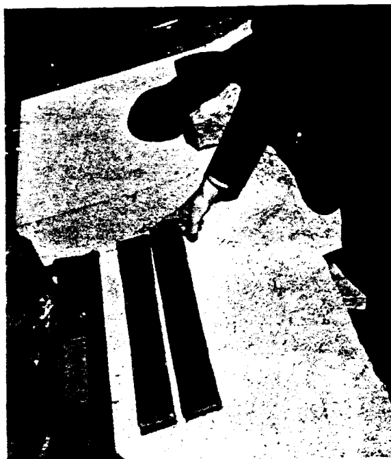
Two views of the lead bearing plates in position on the slope of the pediment and on top of the side walls.
