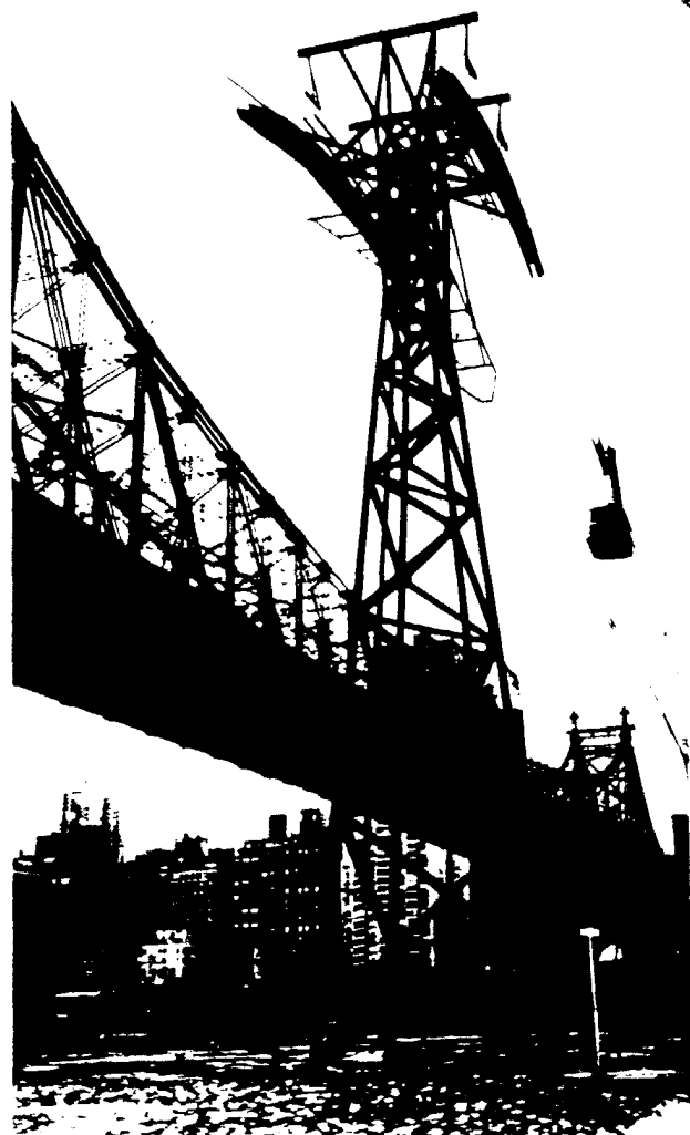
View of tram car as it parallels Queensboro Bridge en route from Manhattan to Roosevelt Island. Lead batteries atop car provide emergency power to run two-way communications equipment and lights for cars.
