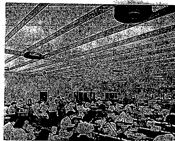
Figure 29. Supplementary lighting provided by adjustable units near the task, which contain two 15-watt fluorescent lamps. A good general lighting system is necessary to provide balanced brightness and a comfortable surround.
