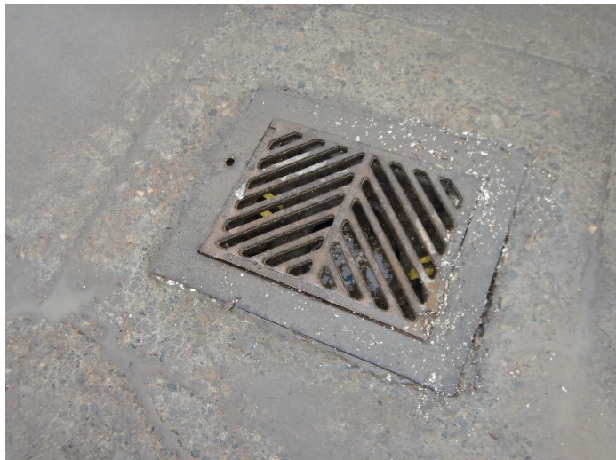
Photo #:41 (DSCN0744) Description: Photo of one of the catch basins.
