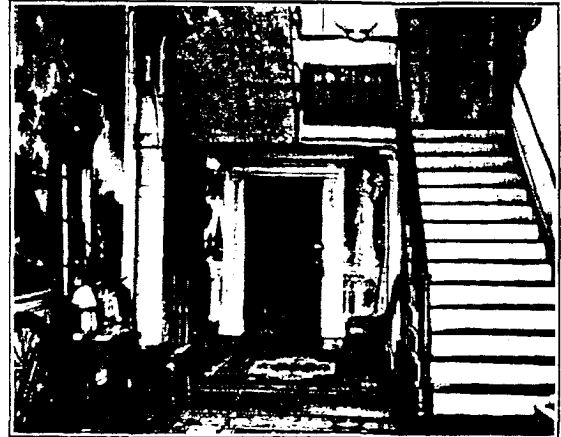
Reception hall at Willow Wall, woodwork painted with pure white lead. Note original furniture and wall-paper.
