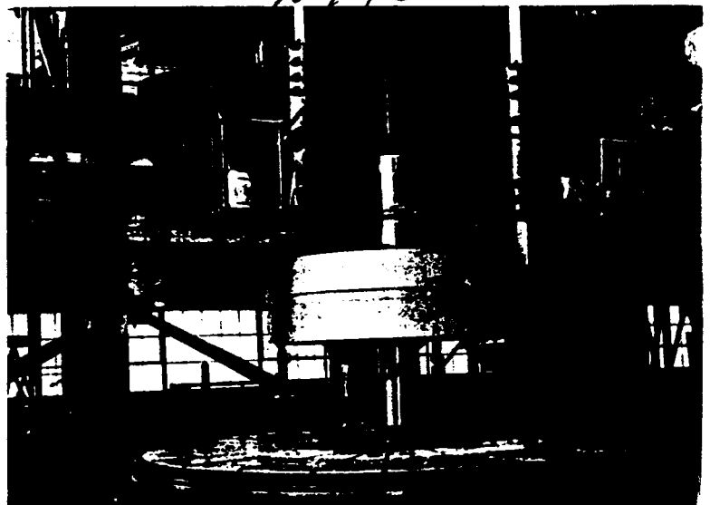
Fig. 10 - Machining a low-speed gear on a 20-ft vertical boring mill at Lynn. This giant and a 14-ft unit have been installed for boring low-speed gear hubs and for turning gear webs and tires.
