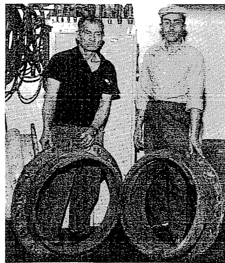
FWT Daniel Cabiroy and Wiper Jose DoVale with the broken expansion joint.
