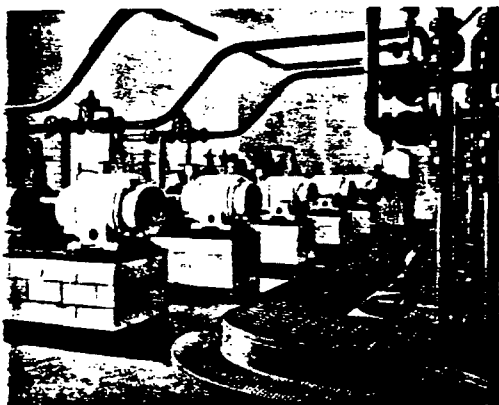
Left, lube blending pumps at the Ponca City refinery not only are kept spotless at all times, but are set up on shiny tile bases. None of the pictures shown has been retouched
