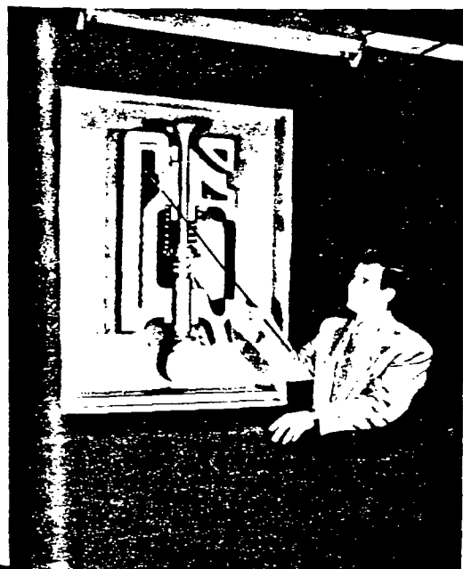
Many of the working models used in the Clinic are 100 times actual size. Here, an oversized exhaust valve is being displayed. The audience is reminded that while car owners often blame gasoline for valve burning, actually this condition usually results from improper seating of the valve
