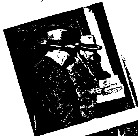
Below, C. W. Butler and V. J. Sittel, of Service Pipe Line, look up the number of a Chicago firm in a telephone directory.
