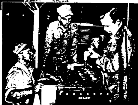
Above, Ethyl engineer Charles Welch shows a Michigan tractor mechanic how to employ a device for determining the valve spring load. Right, use of an electric grinder in proper valve seat reconditioning is demonstrated by Grant Scott, another Ethyl engineer
