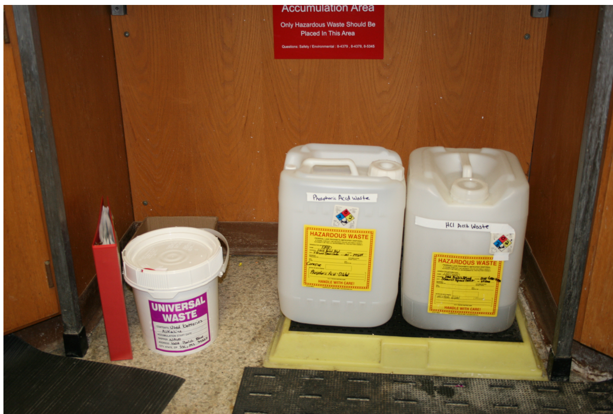
Photo 6 – Building 1003 Room 18 Universal and hazardous waste.
