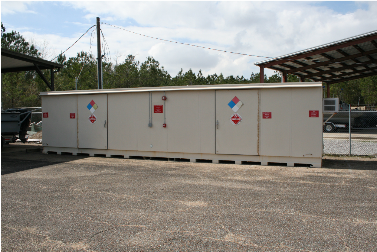
Photo 10 – One of two metal storage buildings located near Building 2408.
