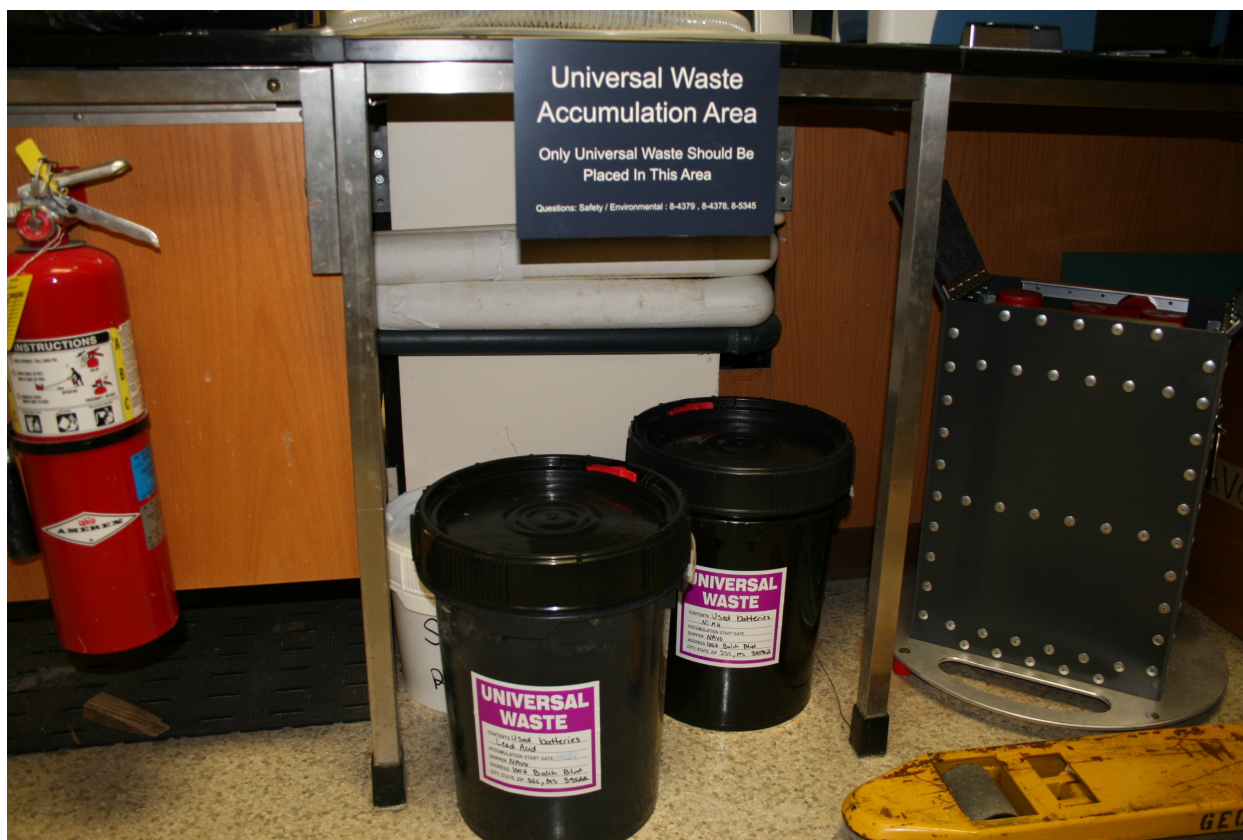
Photo 7 – Building 1003 Room 28 Universal waste batteries.
