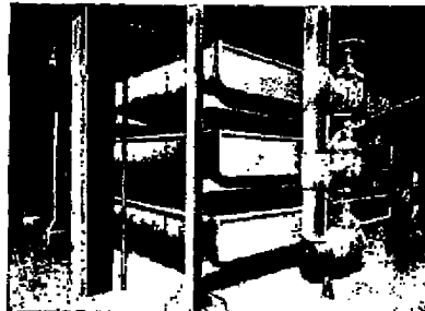
View of pan-room.
