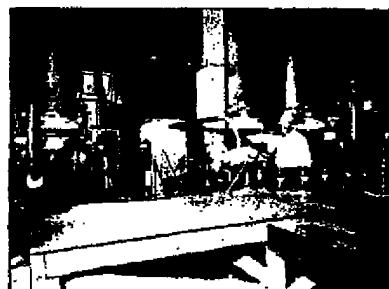
Filling device, where lead is weighed into kegs after being ground in pure refined linseed oil.
