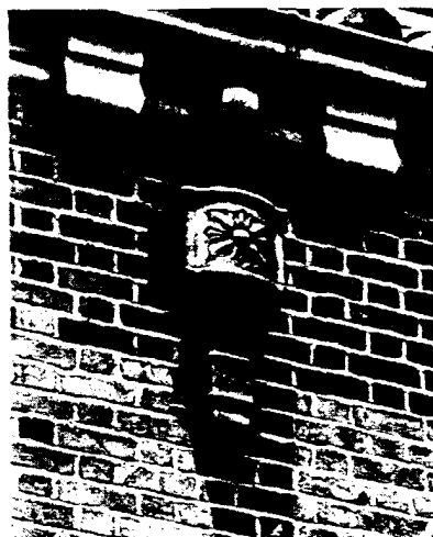
Detail of one of the cast lead ornamental leader-heads.
