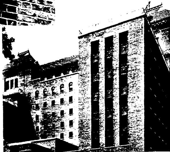
Angle view of the Nurse's Home showing six stories of ornamental lead spandrels on one side.
