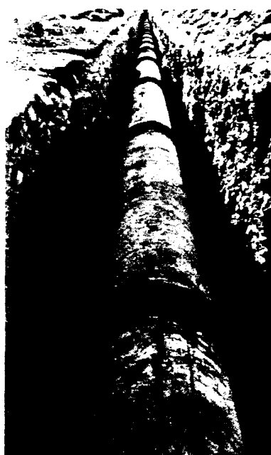
Typical cast iron water main on which lead calking makes watertight, flexible and durable joints
