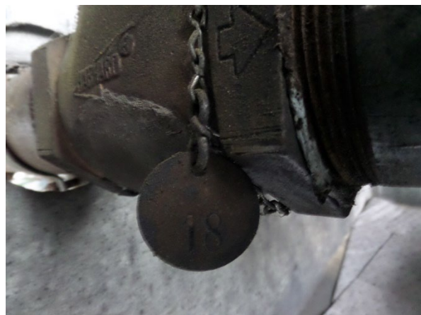
Figure 18: 11:53 AM Tank Farm
