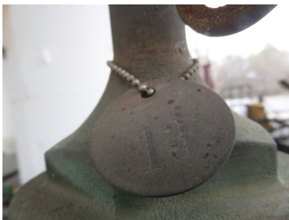
Figure 22: 11:54 AM Tank Farm
