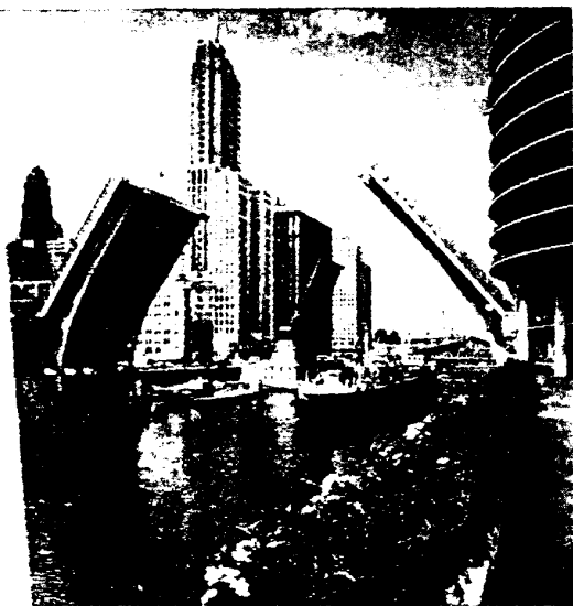
CHICAGO'S NORTH DEARBORN STREET BRIDGE. "It solves the problem of the bascule bridge in a very simple manner."
