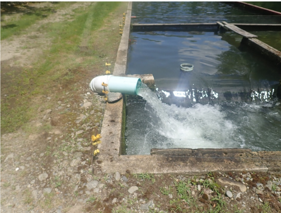
Photo 5. Unpermitted raceways discharging to main raceway series just before outlet to settling ponds and discharge point.
