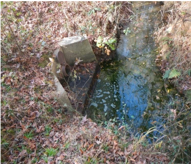
Photo 11. Effluent at outfall was gray in color.
