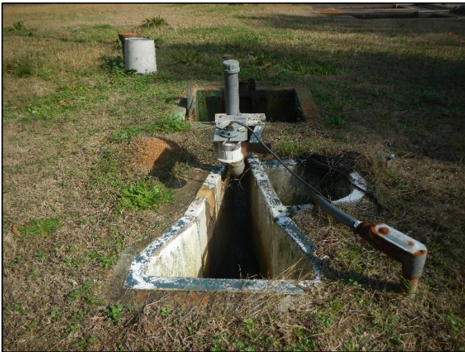
Photo 3. Effluent flowing through the Palmer Bowlus Flume.
