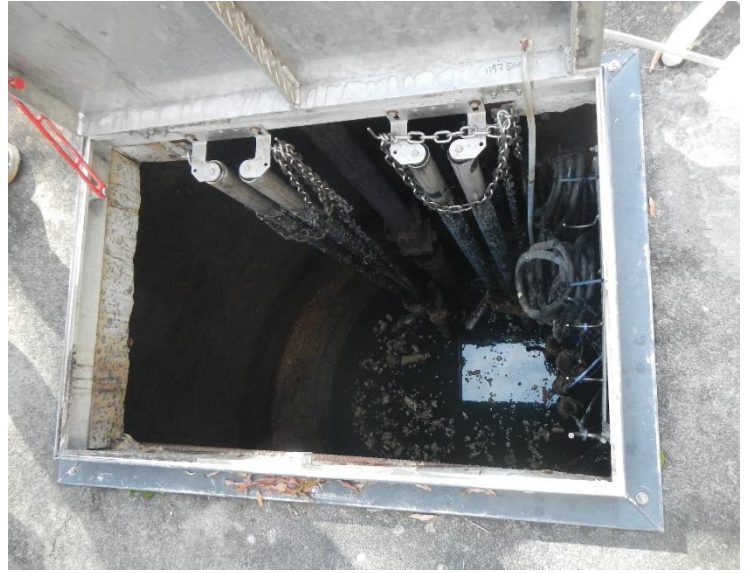
Photo 2. Both influent submersible pumps were operational.
