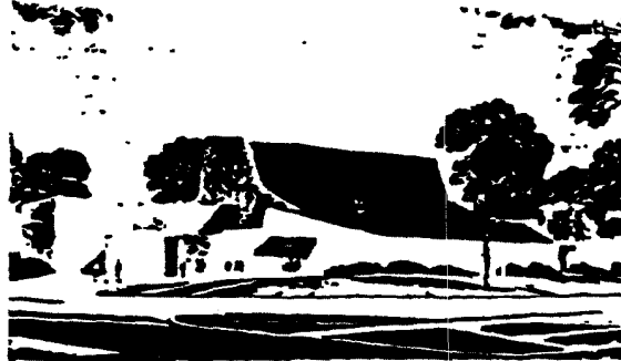
A lead roof shields the drama center from jet roar. The roof is secured strictly under a major air corridor.
