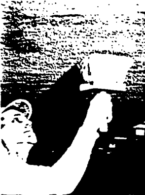
Stippling HI-LITE Acoustical Plaster
