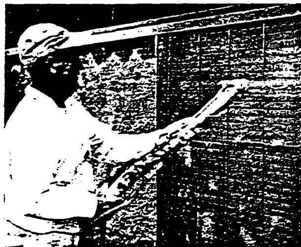
Spraying portland cement base for ORIENTAL Exterior Stucco
