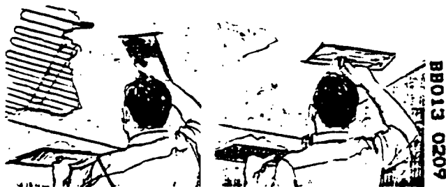
Application of fill coat
