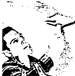
Perforating is done after stippling
