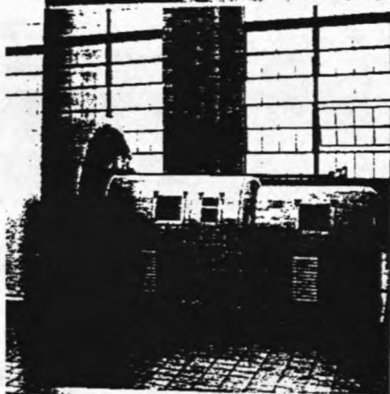
This is how the Piqua turbine room looks at present with the 10,000-kw unit in the foreground followed by the 1000-kw noncondensing unit, a 7500-kw unit installed in 1936, and three 4000-kw units which went into operation in 1934 and 1939.
