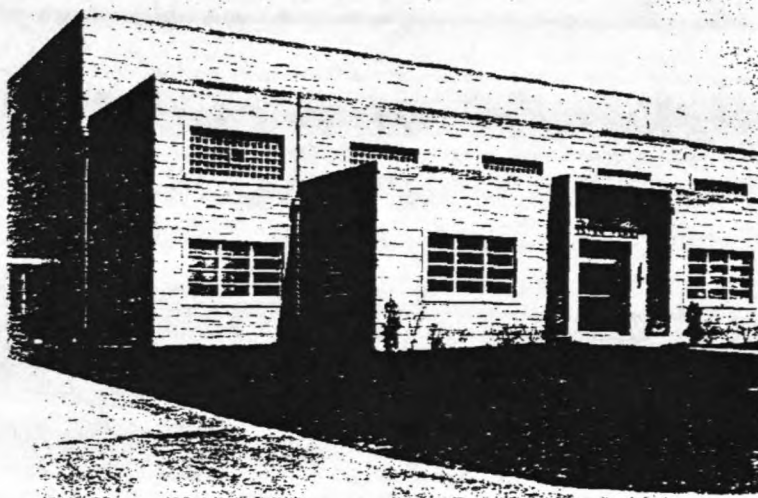
All of the plant's filtering and pumping operations are controlled from the main control panel which is located in this attractive stone building overlooking the dam.
