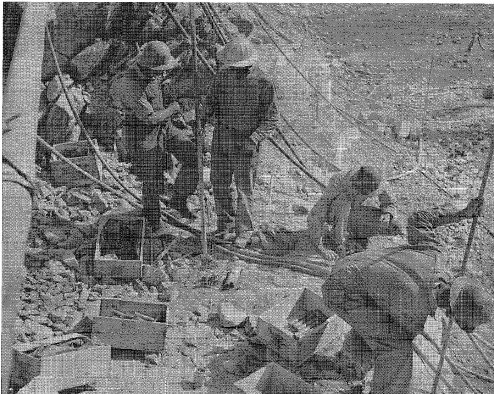
Light, strong air hose made of rayon cord is welcome at construction jobs like this.
