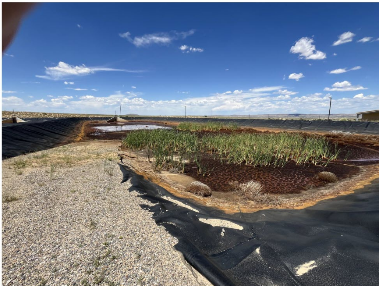
View of the solids drying beds. Note: The dried sludge material is transported and disposed at a landfill. (IMG_0046) (July 10, 2024: 2:40 PM) Photographed by D. Esparza
