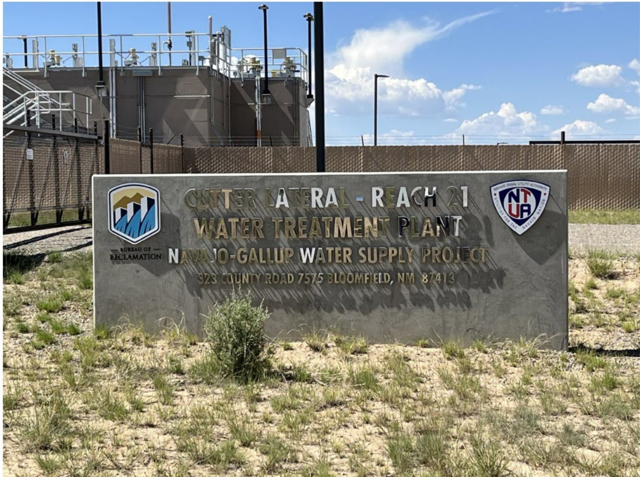
Entrance sign to Cutter Lateral Water Treatment Plant. (IMG_0058) (July 10, 2024: 3:40 PM) Photographed by D. Esparza
