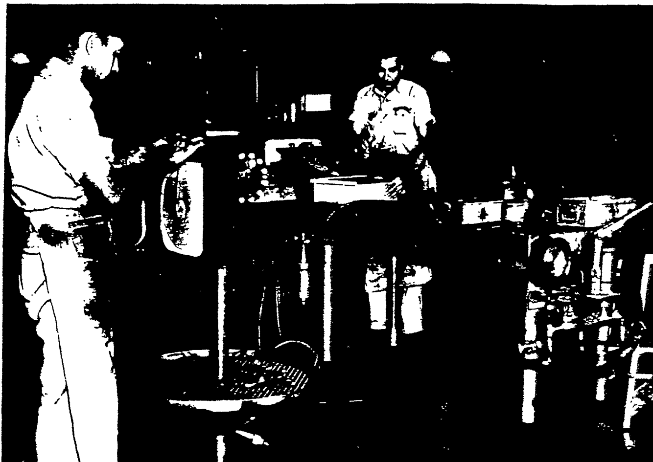
Mercury collection traps used in repairing meters at the Baytown Refinery instrument shops protect employee health.
